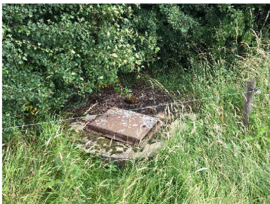
Photo 9: Manhole cover in north east corner of Field 2
