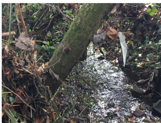
Photo 8: Main Drain, downstream culvert in the northern corner of Field 4
