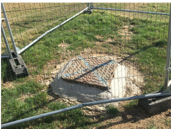
Photo 5: View of manhole in centre of - Field 4
