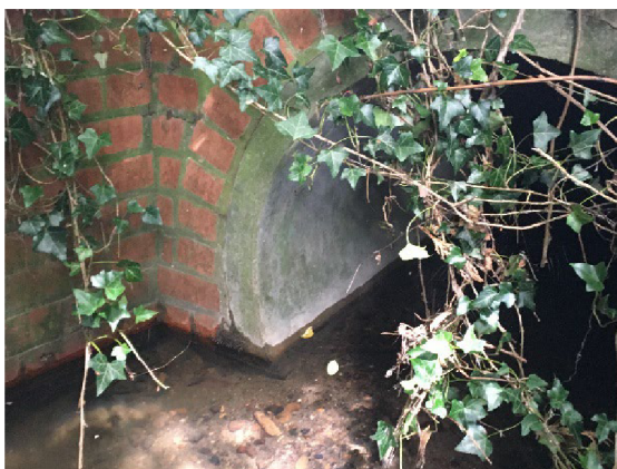
Photo 7: View of Surface Water Sewer entering land drain in south west corner of Field 4
