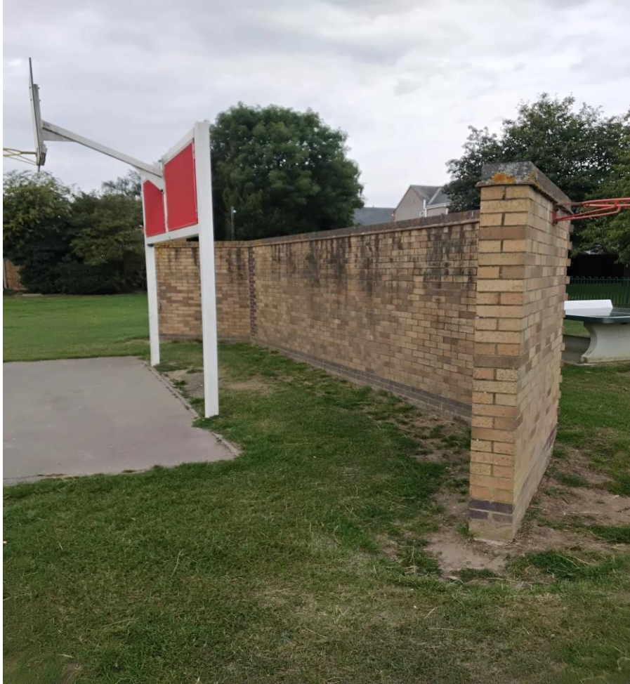
Photo 3. Brick wall on the Site
