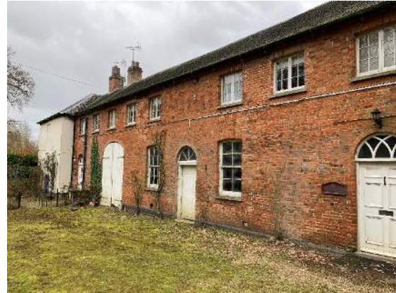
Stable Block – South Elevation
