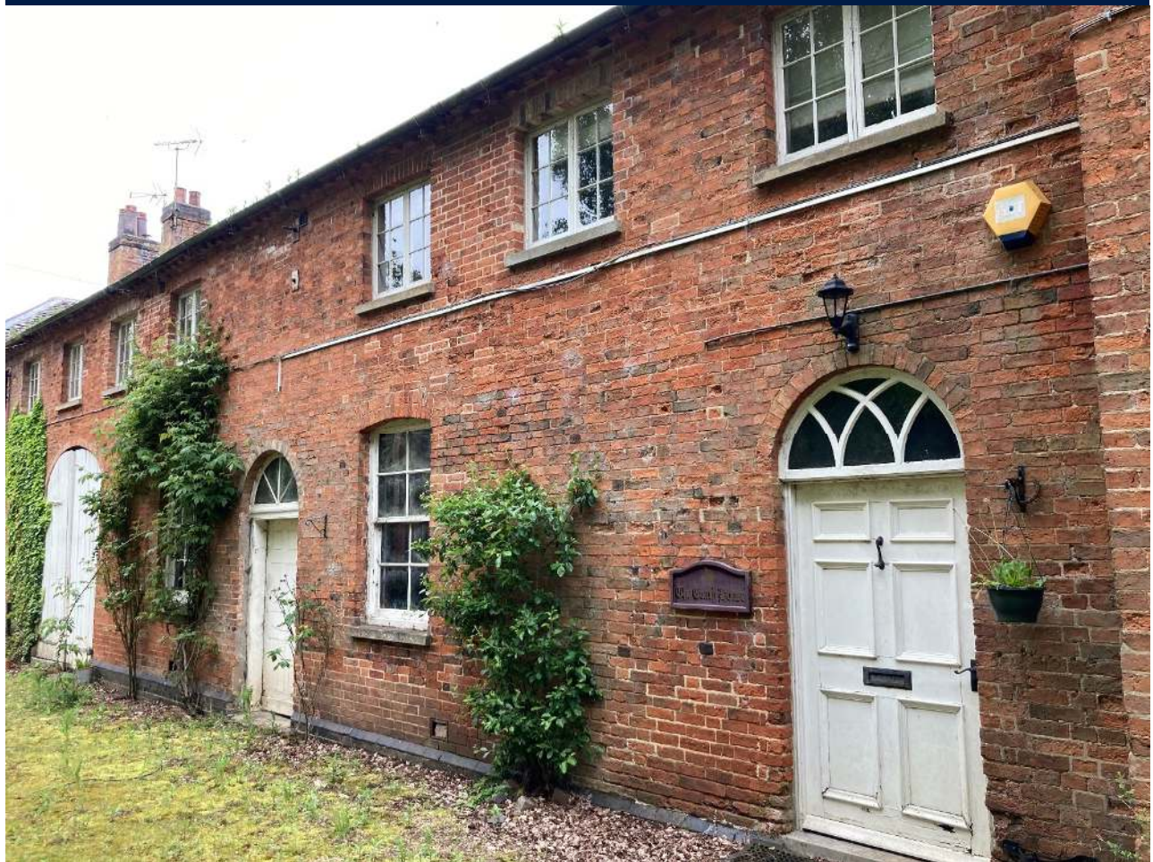
Figure 1. Stable Block, South Elevation (Savills: 2024).
