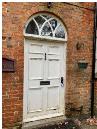
Figure 26. Coach House, entrance door to be retained (Savills: 2024)
