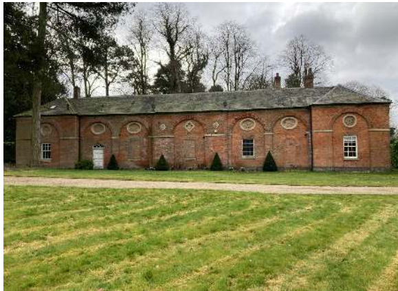
Figure 8. Stable Block, north elevation (Savills, 2024)
