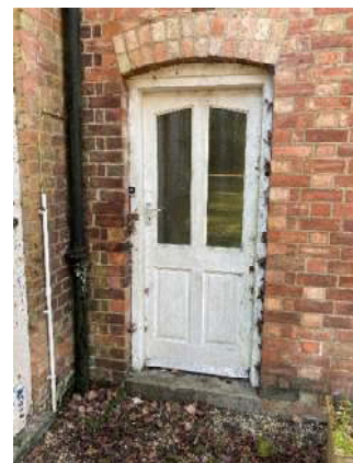
Figure 27. Cottage, modern entrance door (Savills: 2024)
