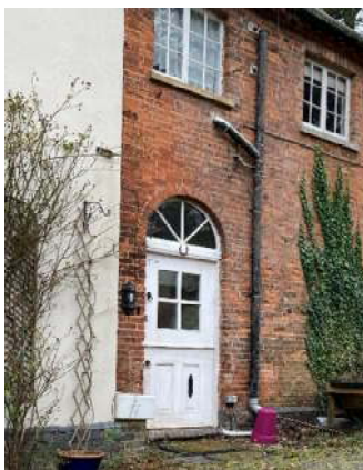
Figure 25. Chauffeur's Cottage, modern entrance door (Savills:2024).
