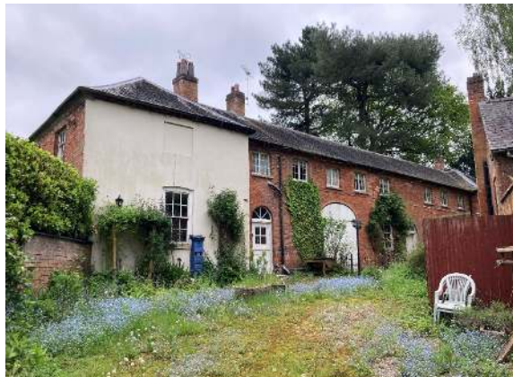
Figure 10. Stable Block, south elevation (Savills, 2024)
