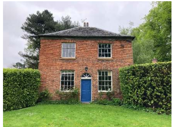
Figure 11. Stable Block, west elevation (Savills, 2024)
