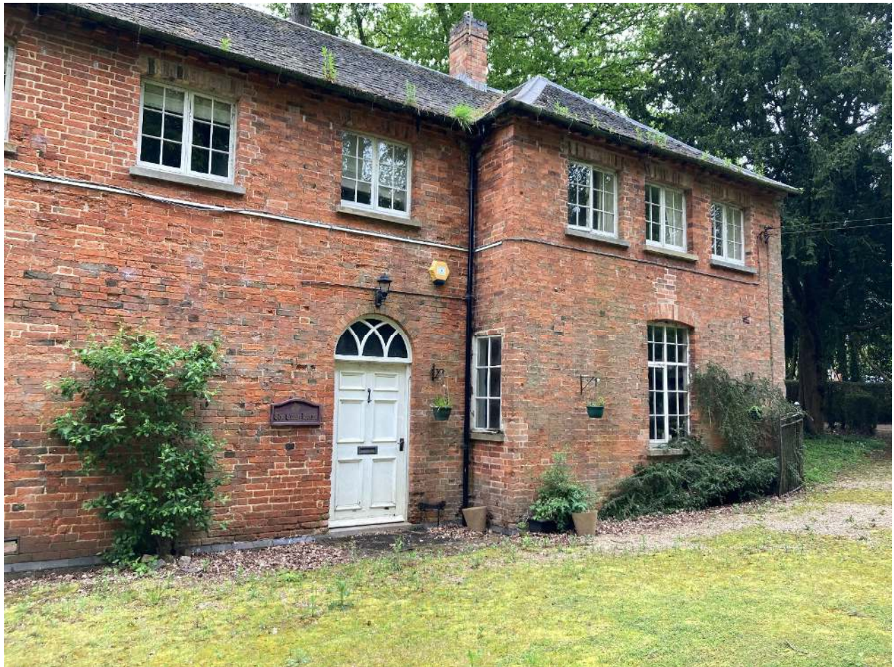
Figure 1. Stable Block, South Elevation (Savills: 2024).
