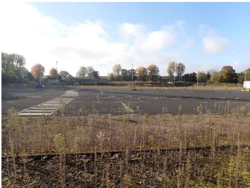
Plate 28: Looking south-west from the northern boundary showing changes in ground level.
