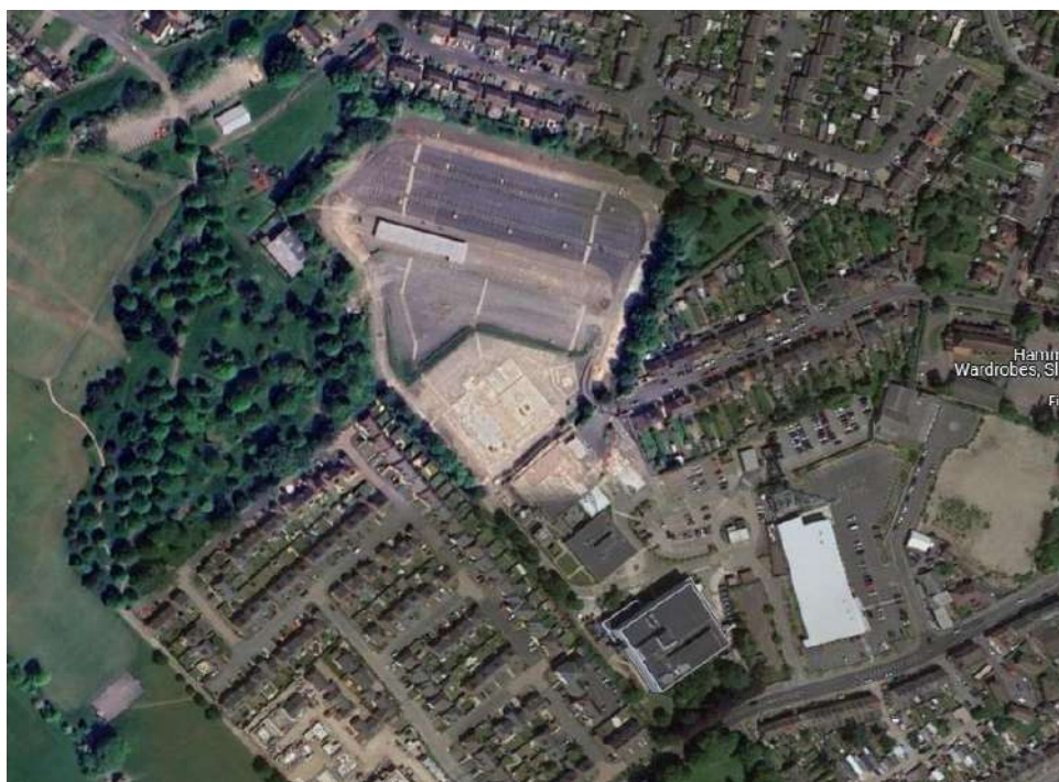
Plate 25 Aerial image showing the locations of the latest phase of development, mainly along the western boundary.
