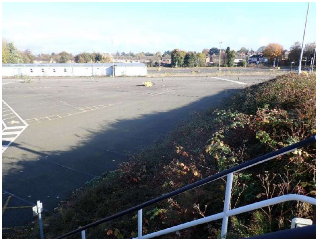
Plate 27: Looking north-east across the northern part of the Site. Note steps down and much lower level.
