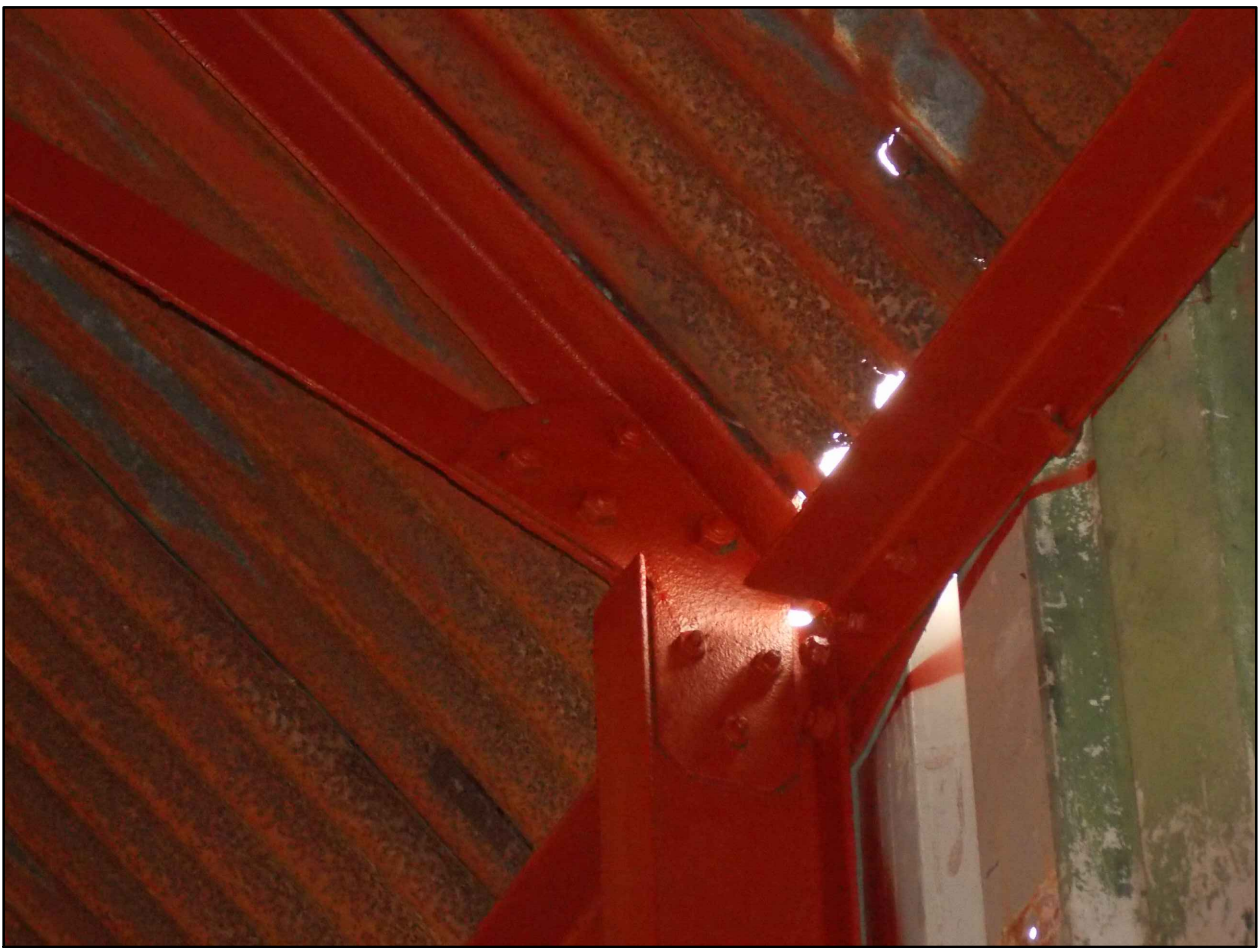
Eaves / truss conection.
