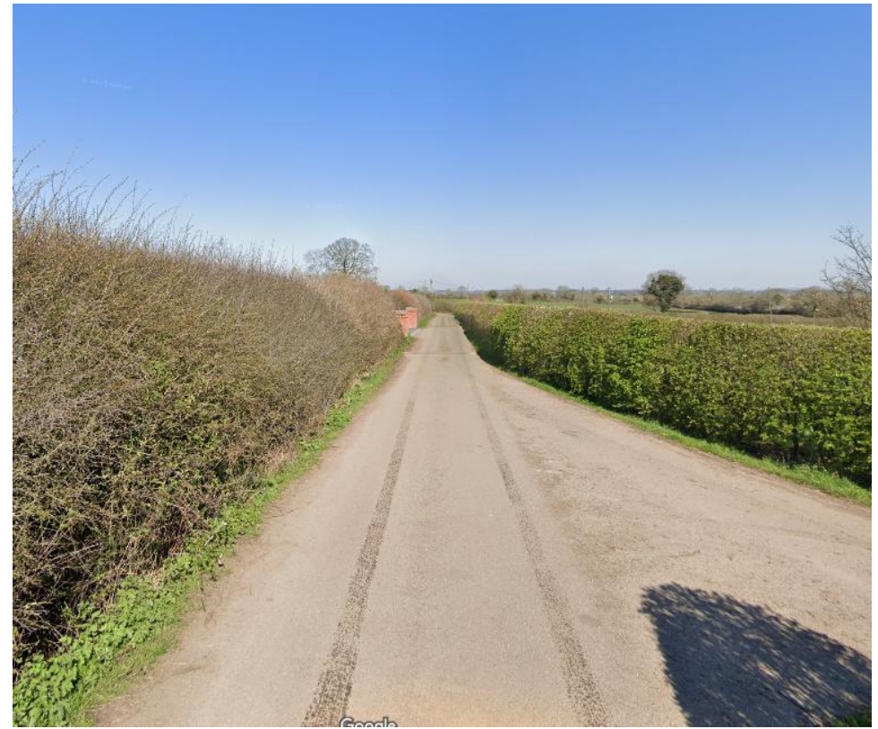
Figure 4. Facing north on unnamed road.
