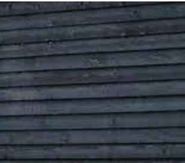
Black stained timber - Frame and Horizontal timber boarding
