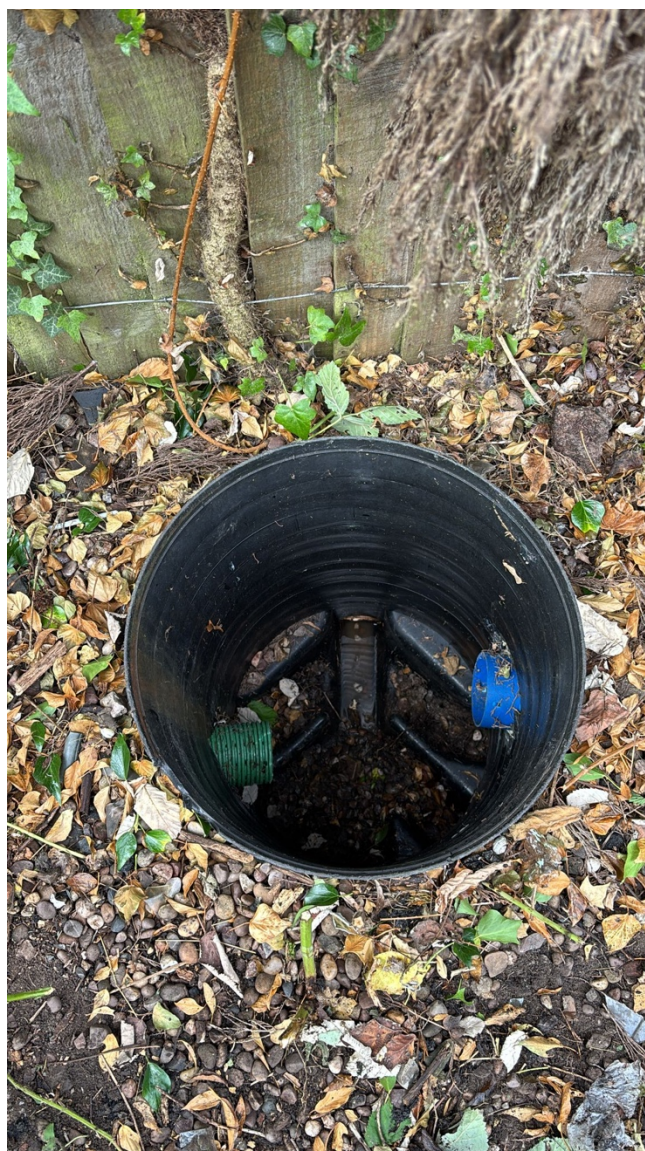
Fig 1 – Existing SW chamber
