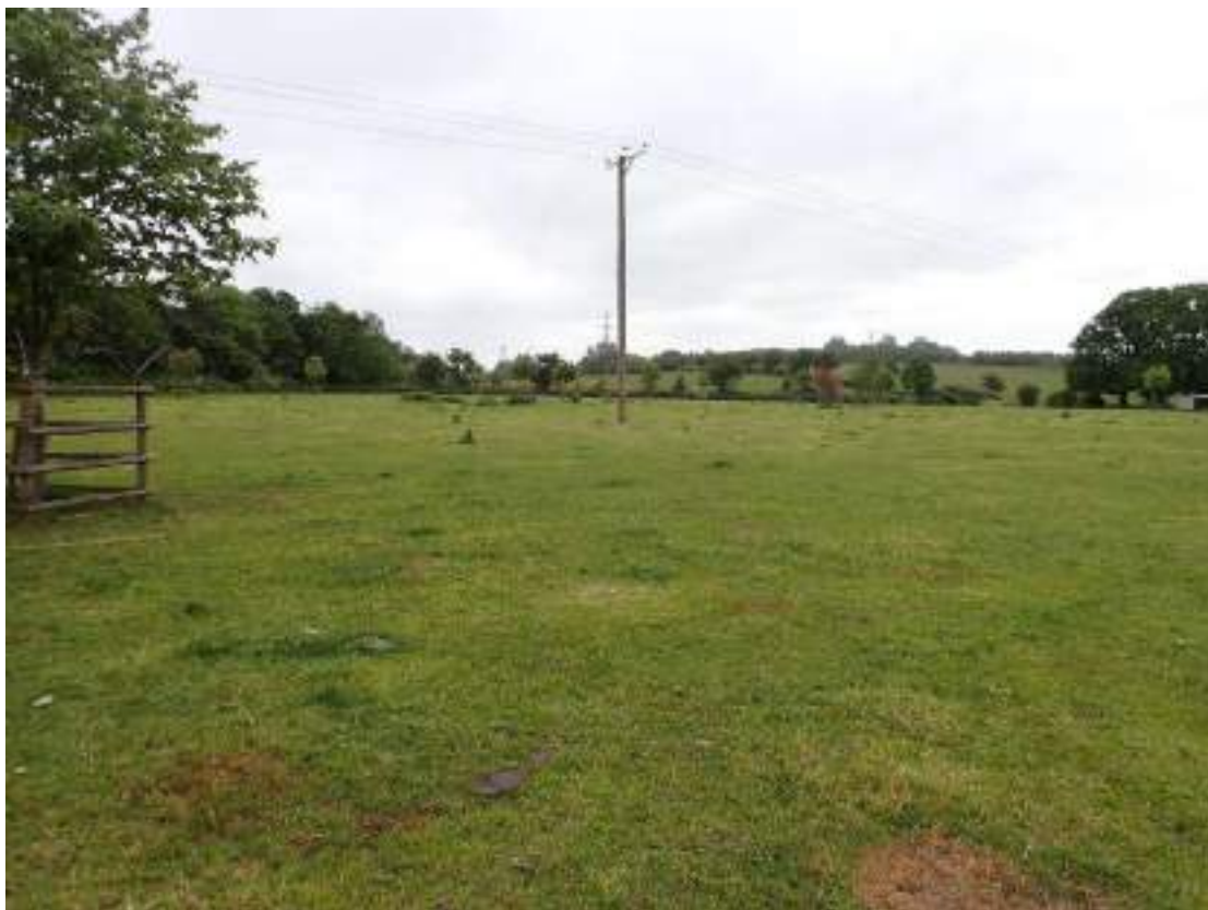
Plate 05: East to West Overhead Service Cable. Field 01.
