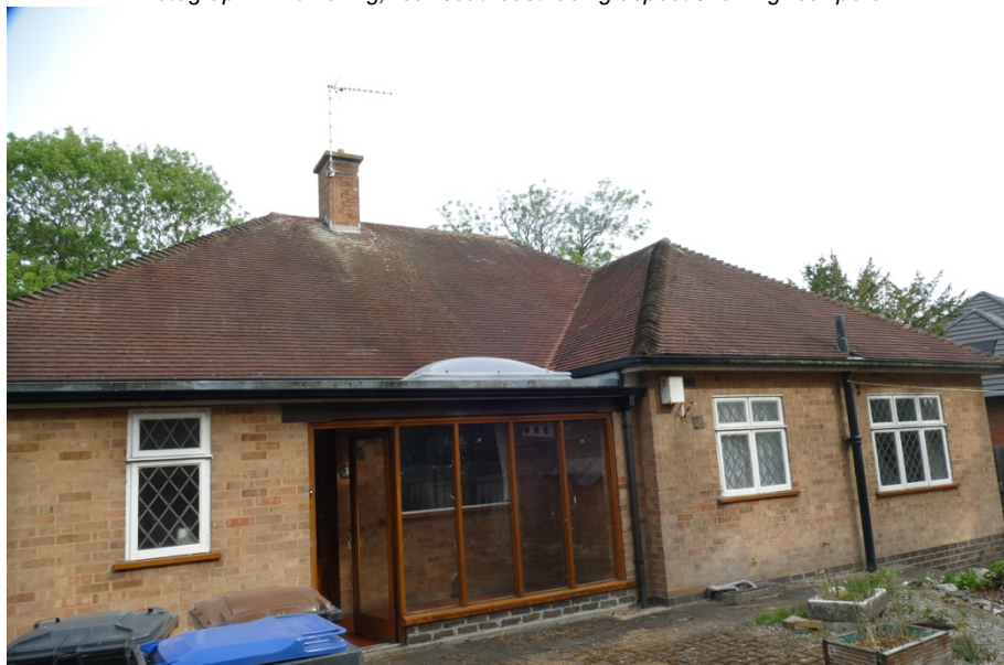
Photograph 2 – dwelling, rear southeast facing aspect showing rear porch.
