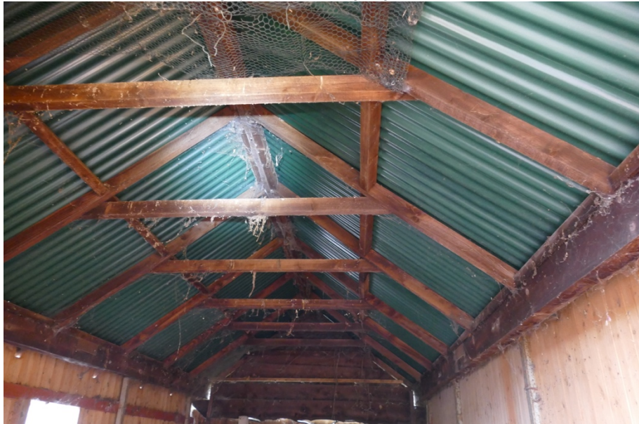
Photograph 6 – detached garage roof detail.
