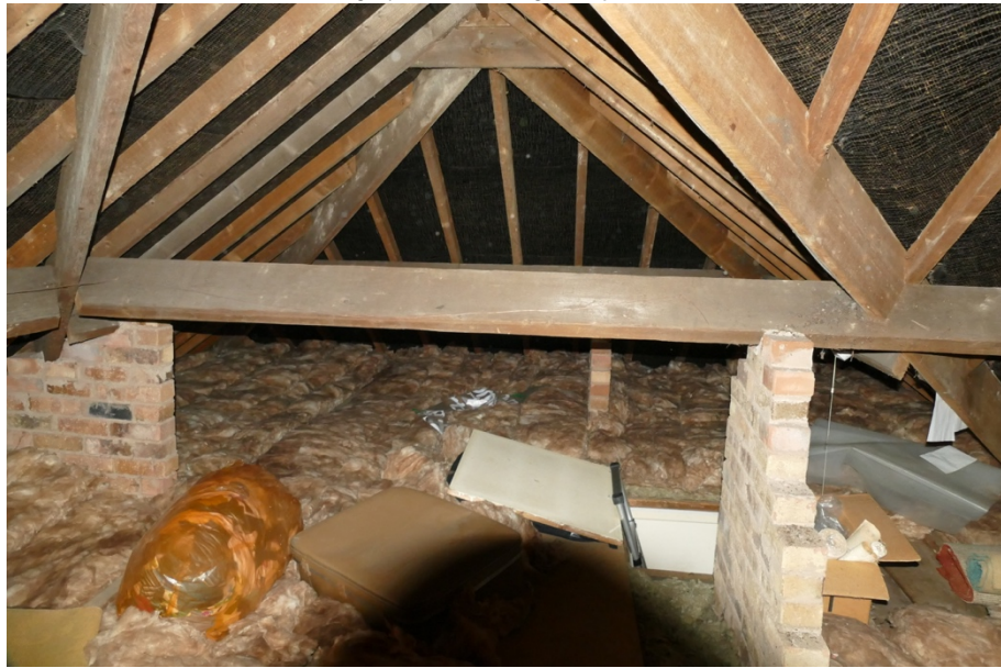
Photograph 5 – dwelling roofspace detail.
