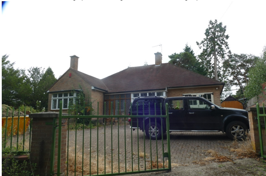
Photograph 1 – dwelling, front, northwest facing aspect.
