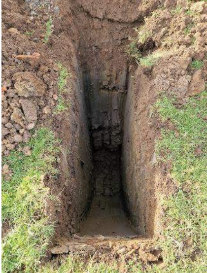
PLATE 41 – Trial Pit Excavation – TP18.
