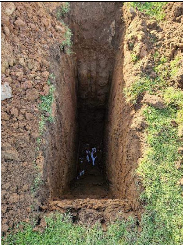
PLATE 39 – Trial Pit Excavation – TP17.
