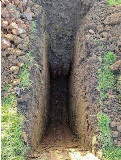
PLATE 35 – Trial Pit Excavation – TP15.
