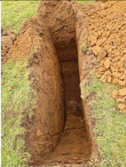
PLATE 07 – Trial Pit Excavation – TP01.
