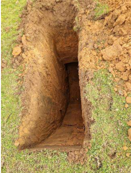
PLATE 09 – Trial Pit Excavation – TP02.
