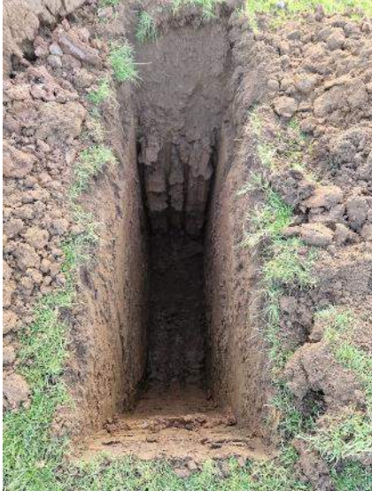
PLATE 33 – Trial Pit Excavation – TP14.
