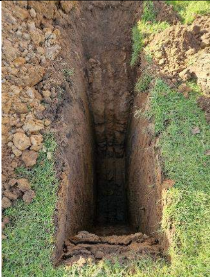
PLATE 31 – Trial Pit Excavation – TP13.
