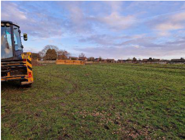
PLATE 01 – Site Overview – Looking North.
