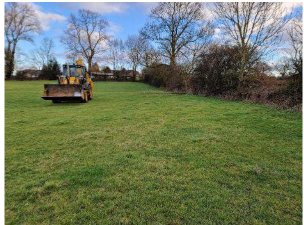
PLATE 04 – Site Overview – Looking North.
