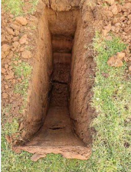
PLATE 29 – Trial Pit Excavation – TP12.
