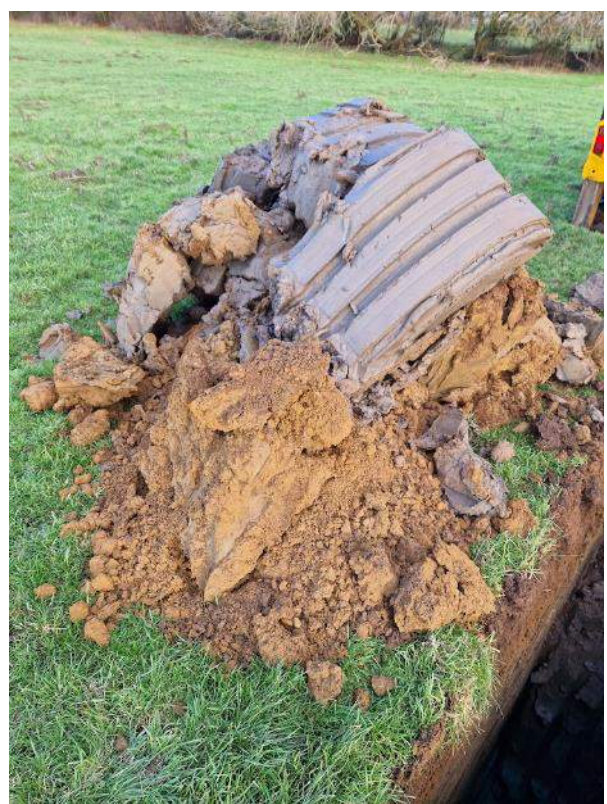
PLATE 52 – Trial Pit Spoil – TP23.
