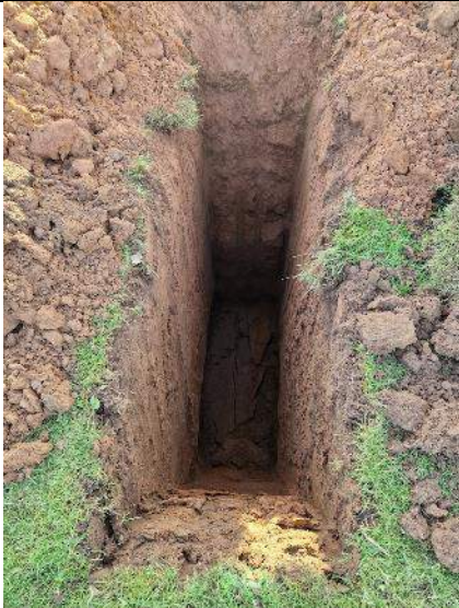
PLATE 43 – Trial Pit Excavation – TP19.
