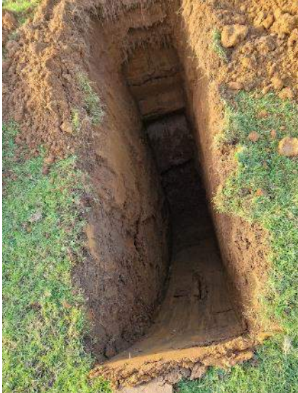
PLATE 15 – Trial Pit Excavation – TP05.
