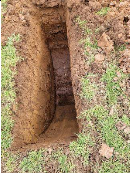
PLATE 19 – Trial Pit Excavation – TP07.
