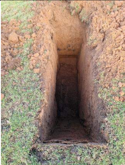
PLATE 23 – Trial Pit Excavation – TP09.
