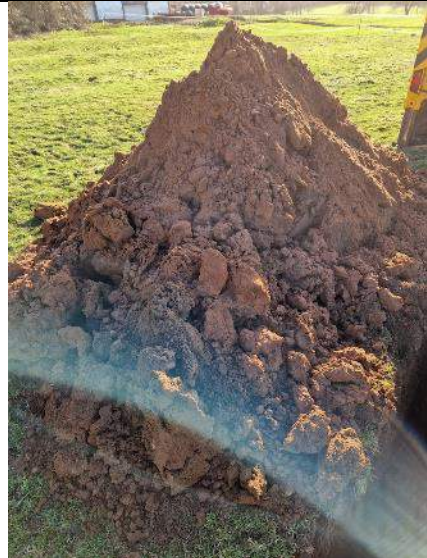
PLATE 48 – Trial Pit Spoil – TP21.
