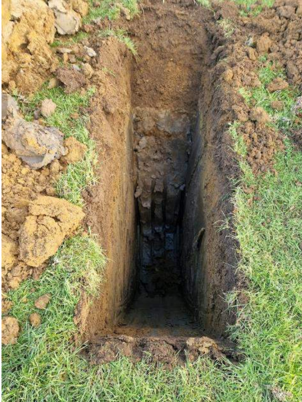
PLATE 51 – Trial Pit Excavation – TP23.
