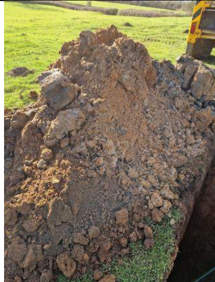
PLATE 32 – Trial Pit Spoil – TP13.
