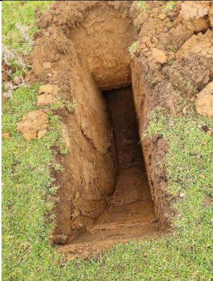
PLATE 27 – Trial Pit Excavation – TP11.
