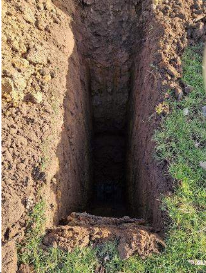
PLATE 45 – Trial Pit Excavation – TP20.
