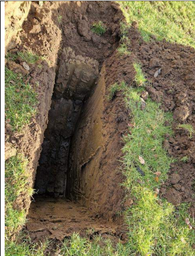
PLATE 53 – Trial Pit Excavation – TP24.
