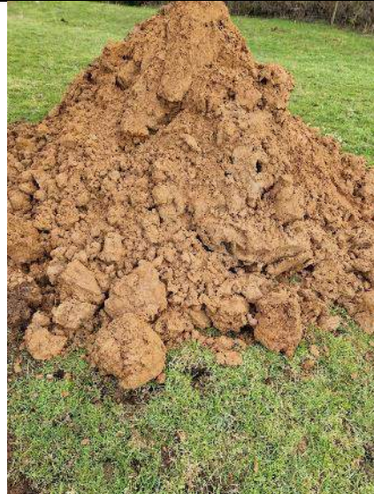
PLATE 28 – Trial Pit Spoil – TP11.
