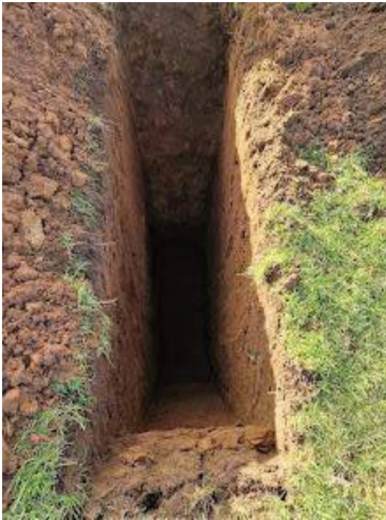
PLATE 37 – Trial Pit Excavation – TP16.
