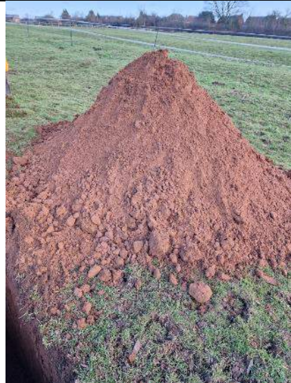
PLATE 24 – Trial Pit Spoil – TP09.
