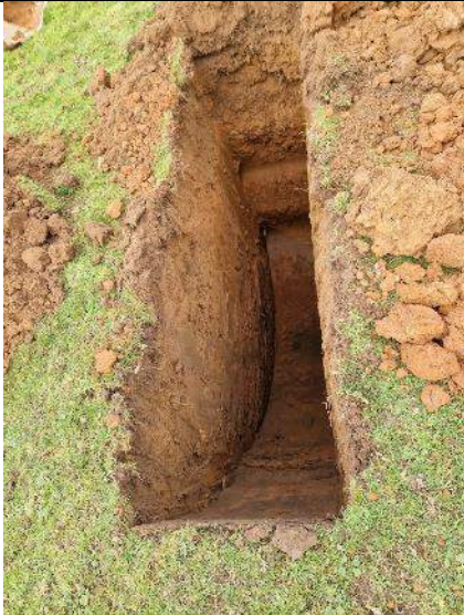
PLATE 11 – Trial Pit Excavation – TP03.
