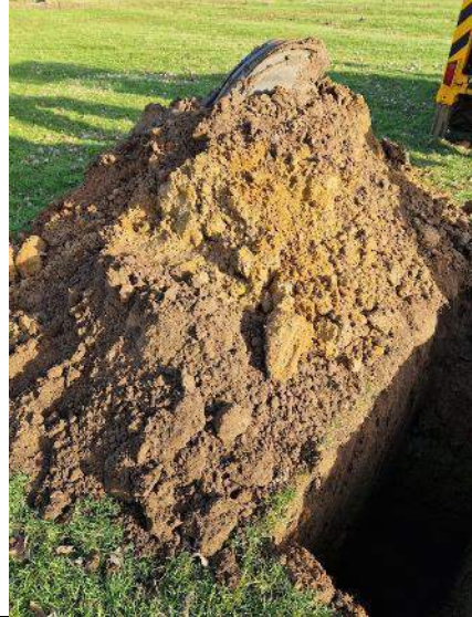
PLATE 46 – Trial Pit Spoil – TP20.
