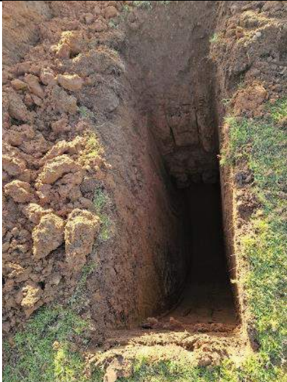
PLATE 47 – Trial Pit Excavation – TP21.
