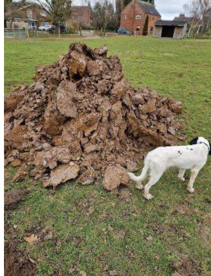
PLATE 14 – Trial Pit Spoil – TP04.
