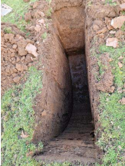
PLATE 25 – Trial Pit Excavation – TP10.
