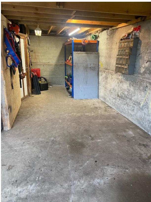
Photograph 2 – Mezzanine floor to right hand end of barn
