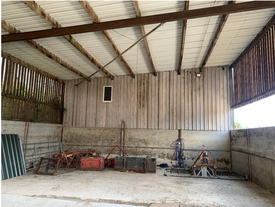
Photograph 1 – Internal view of left hand side of barn
