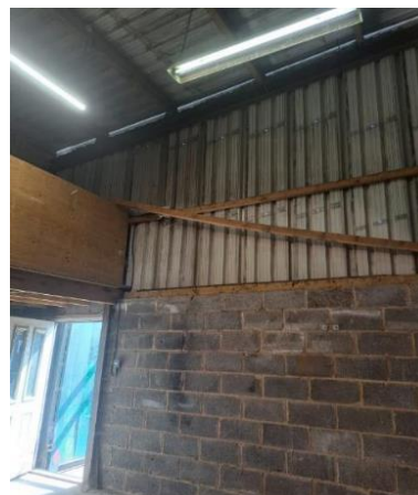
Photograph 4: walls within Barn 2.
