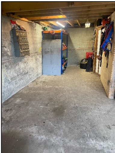
Photograph 5: interior of Barn 2.
