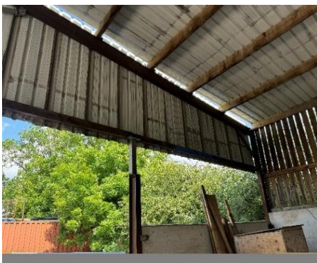
Photograph 3: Open end in Barn 1 at western elevation.
