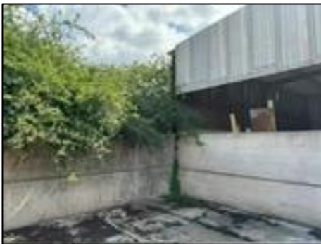
Photograph 1: Barn 1 from outside.
