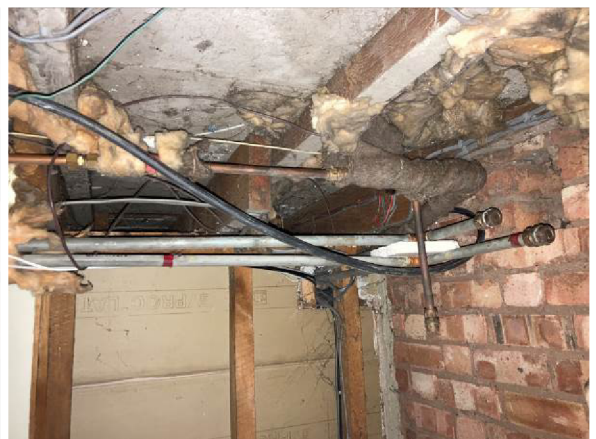
Small loft interior (south end of roof)
