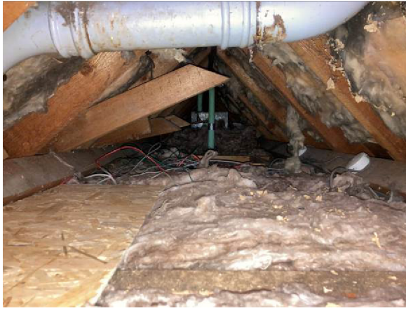
Small loft in north western roof
