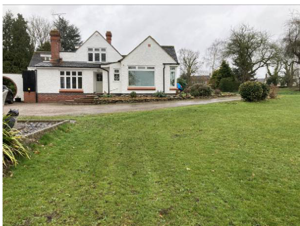
Lawn to the north west side of the house
