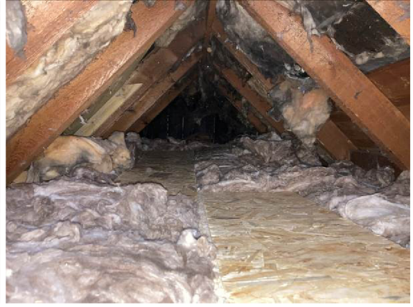
Small loft in north western roof
