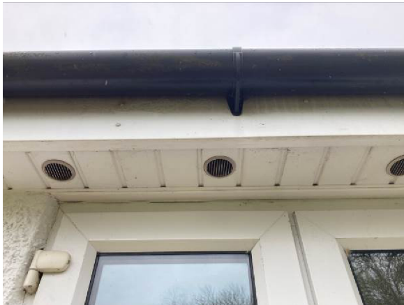
Close up of uPVC roof edge
