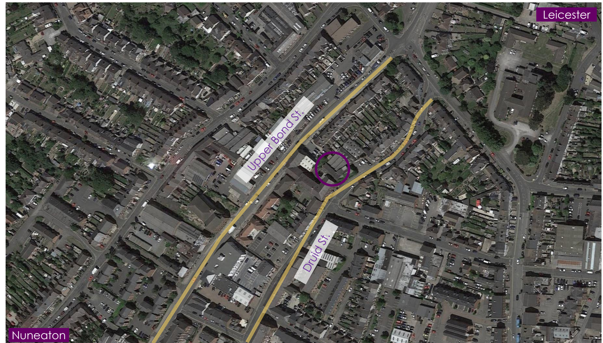
Aerial view of the site with the Laban Tansey building highlighted
