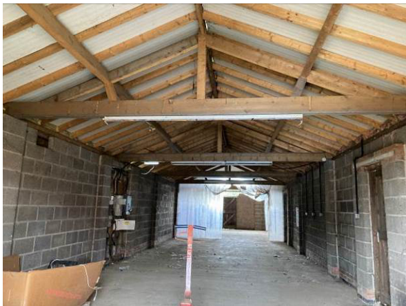
Interior of B4
