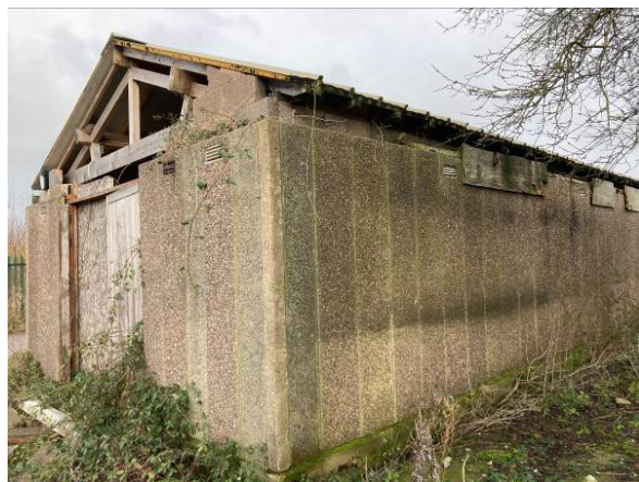
Exterior of B4 east end
