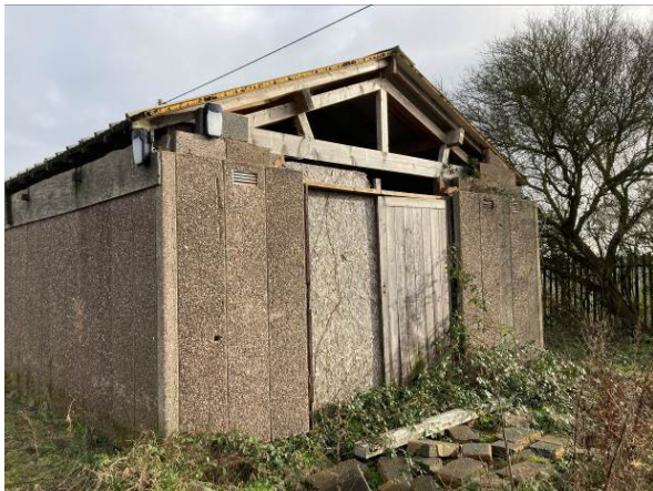
Exterior of B4 west end
