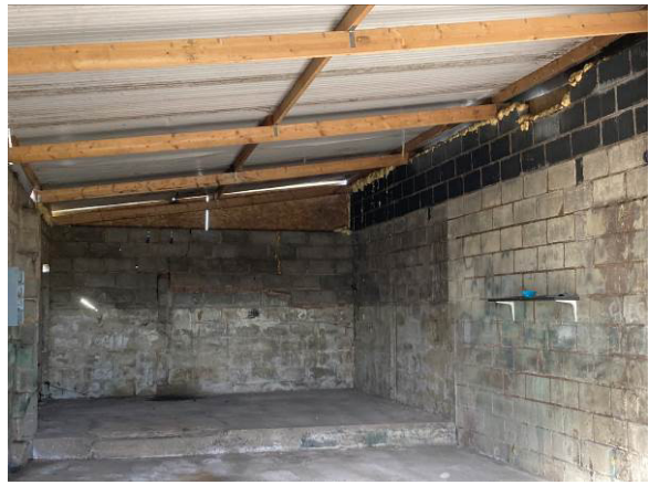
Interior of B3
