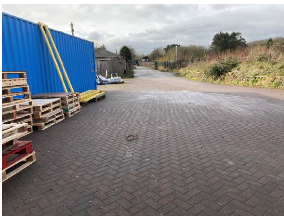
Hardstanding near B2
