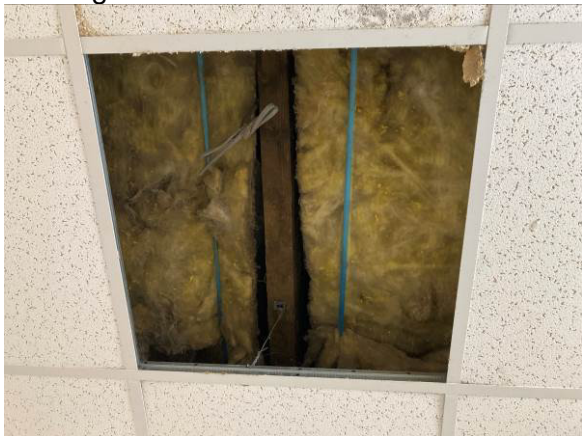
Underside of roof B1
