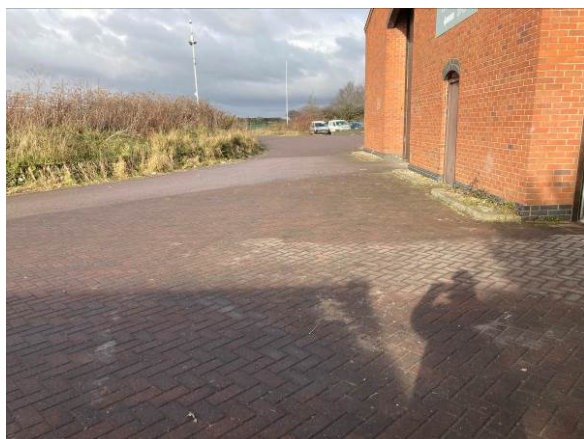
Hardstanding near B2
