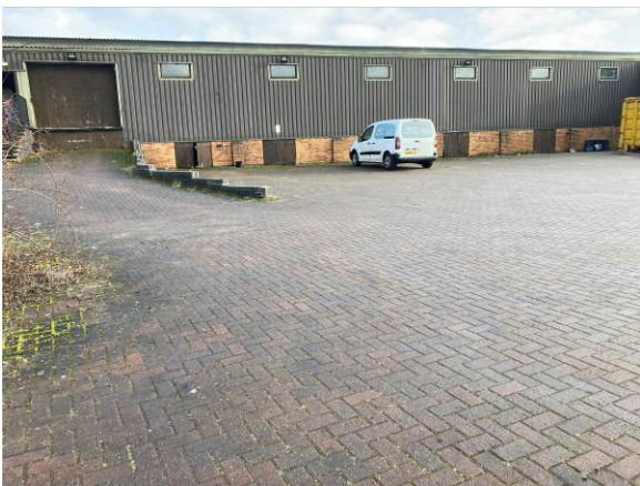
Hardstanding near B1
