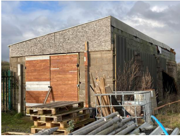
South face of B3
