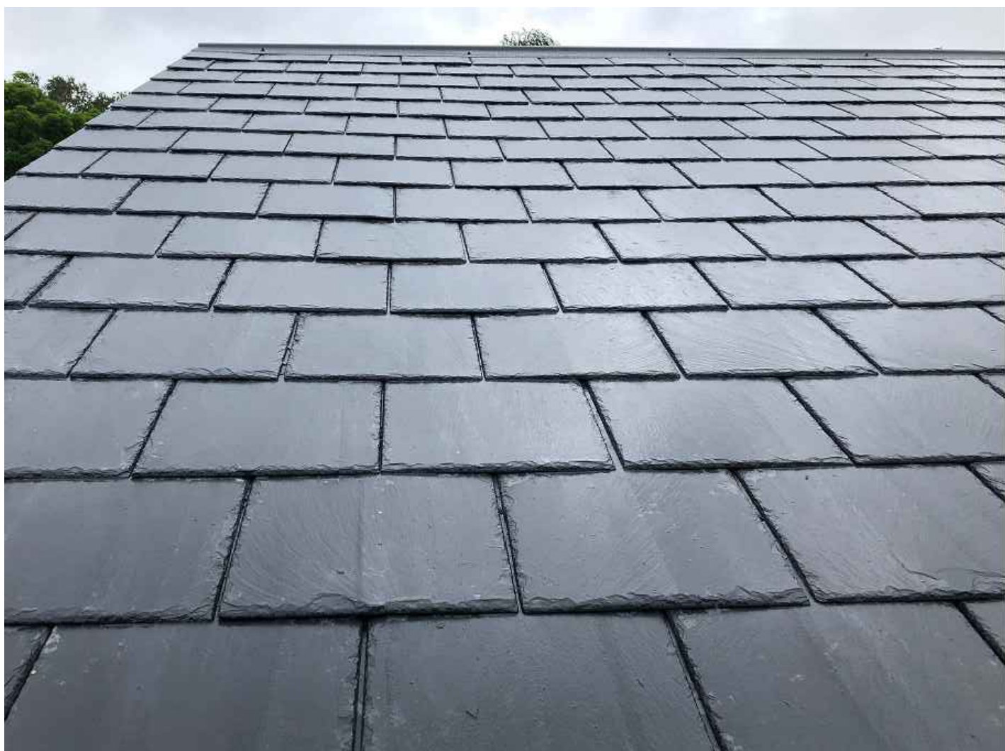
Example Roof Covering
