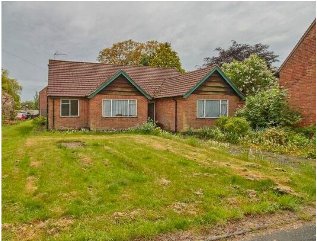
Fig 8. Existing Bungalow before demolition
