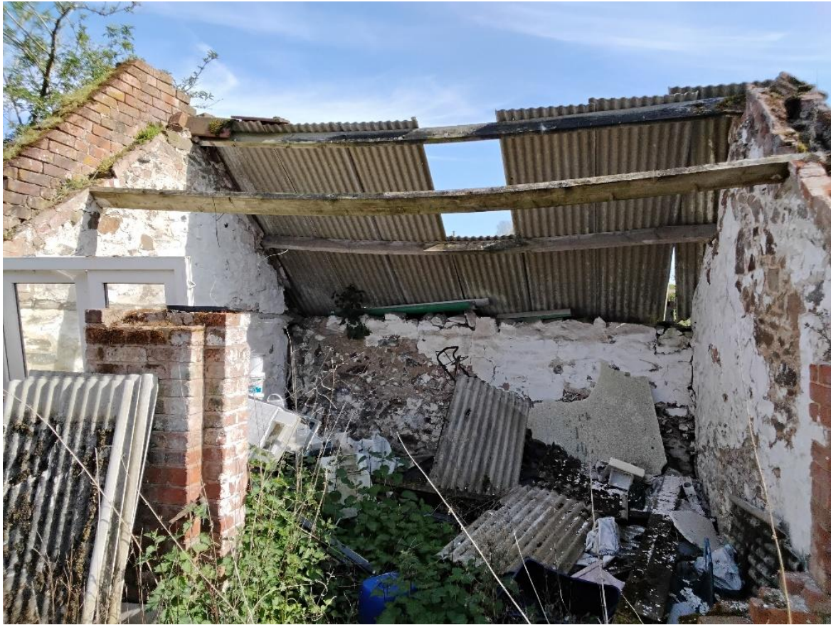
Photo 2. Western cell of the former stable block, with roof still partly intact.
