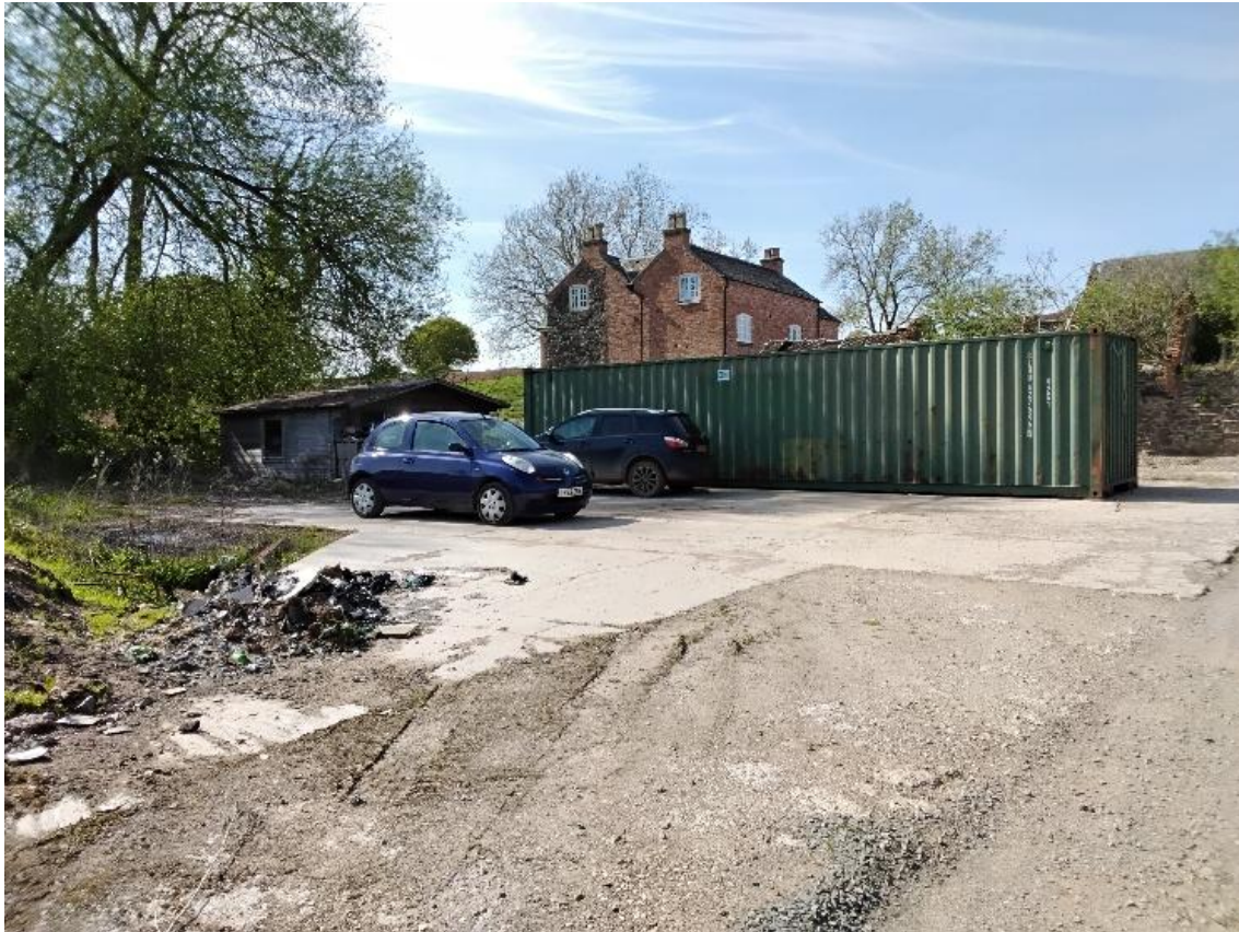
Photo 4. Concrete slab and packed stone and gravel typical of the Site. The encroaching vegetation on the left of the photo is outside of the red line boundary.
