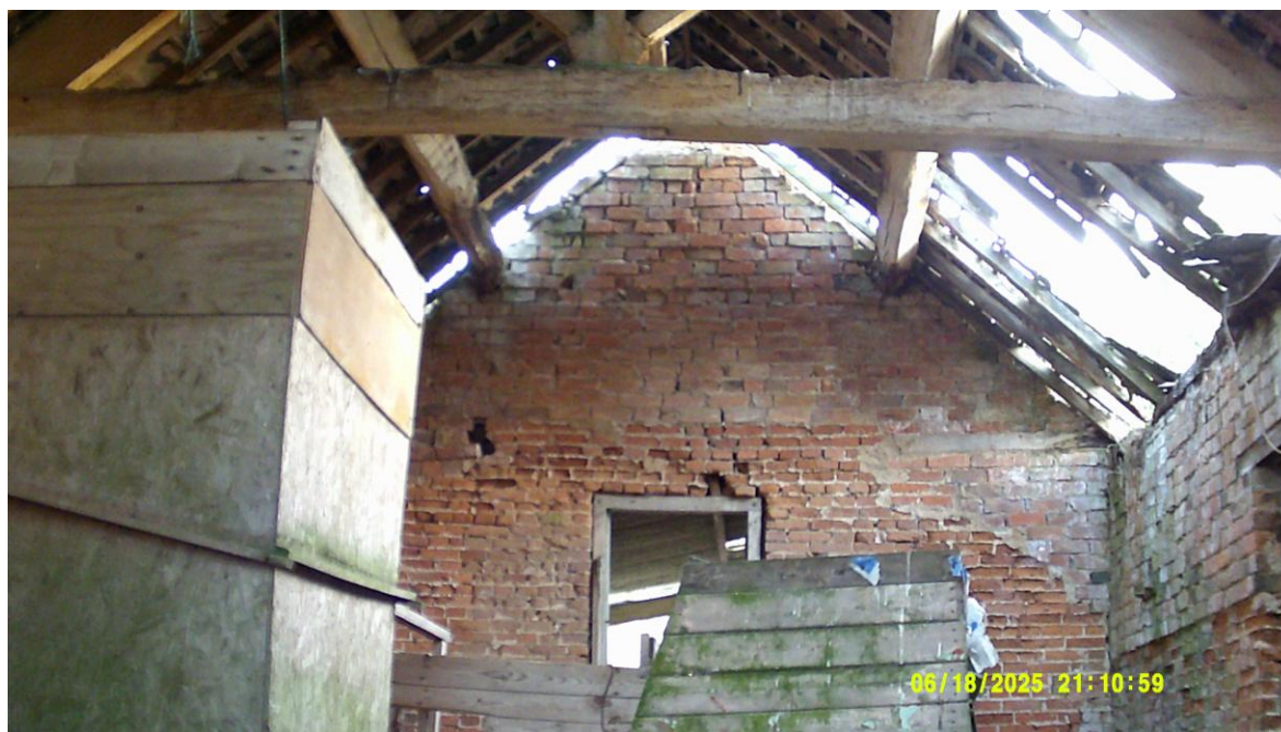
Photo 3: Internal view of the upper floor
