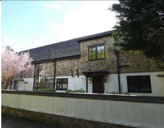
Photograph 1. The western end of the north elevation of the house
