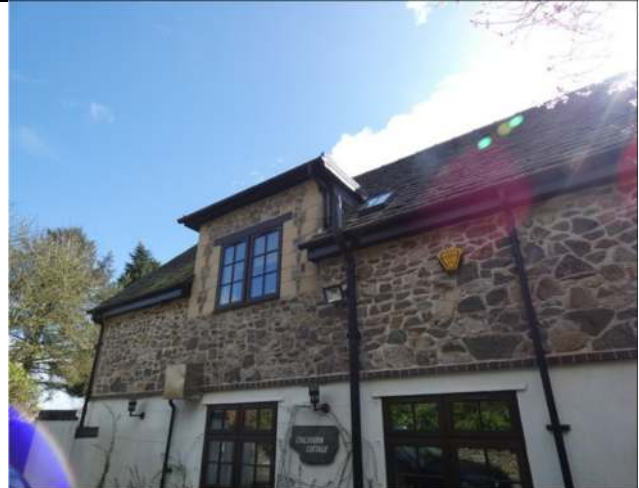
Photograph 2. The eastern end of the north elevation of the house
