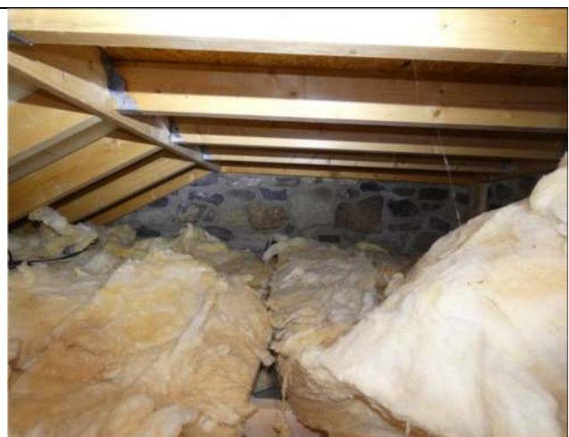
Photograph 30. The enclosed roof void within the single-storey extension at the south-west corner of the house
