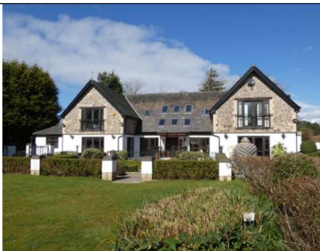
Photograph 5. The south elevation of the house
