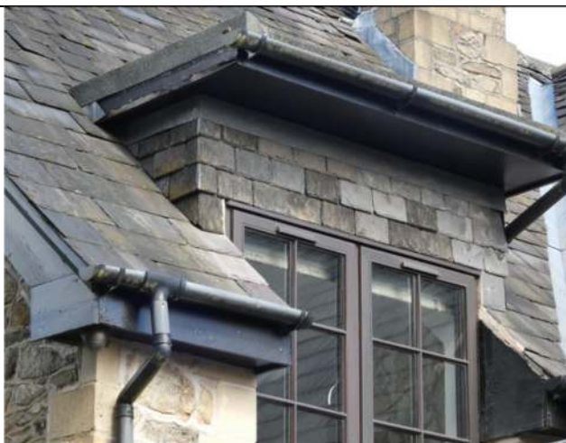
Photograph 11. Example of a dormer window
