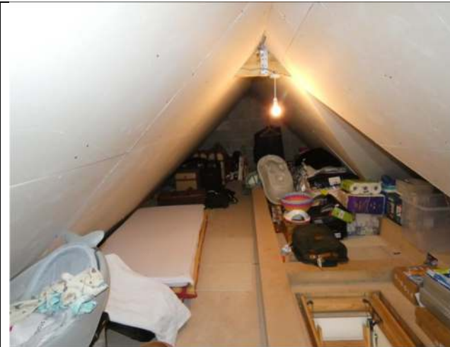
Photograph 25. The eastern section of enclosed roof void within the house (view to east)
