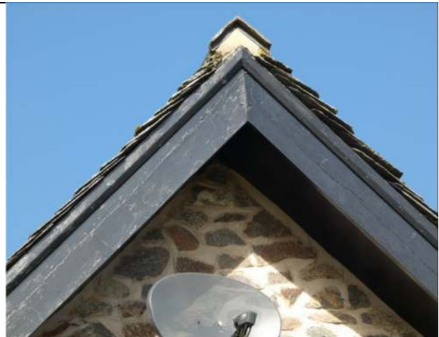
Photograph 16. Example of the soffit and fascia above a gable wall
