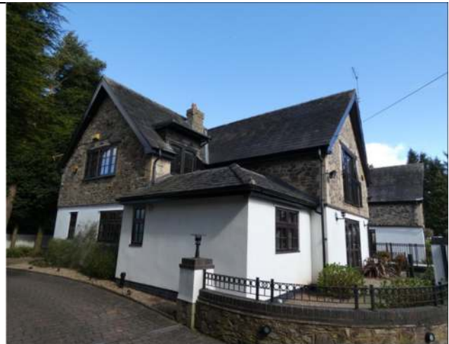
Photograph 4. The west elevation of the house
