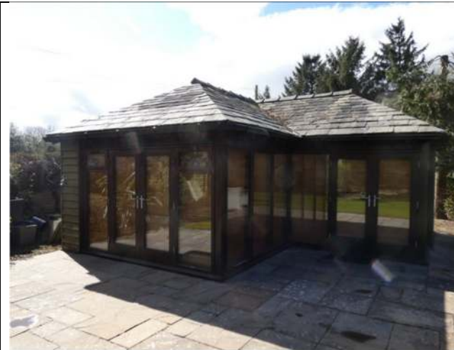
Photograph 31. The east elevation of the outbuilding
