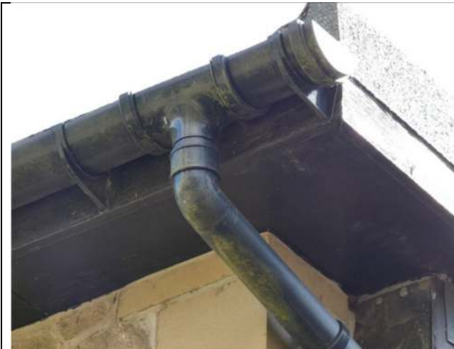
Photograph 15. Example of the soffit and fascia
