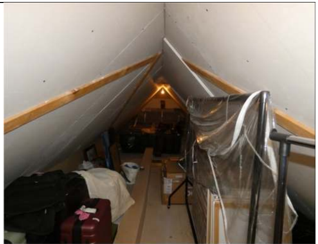
Photograph 22. The western section of enclosed roof void (view to east)
