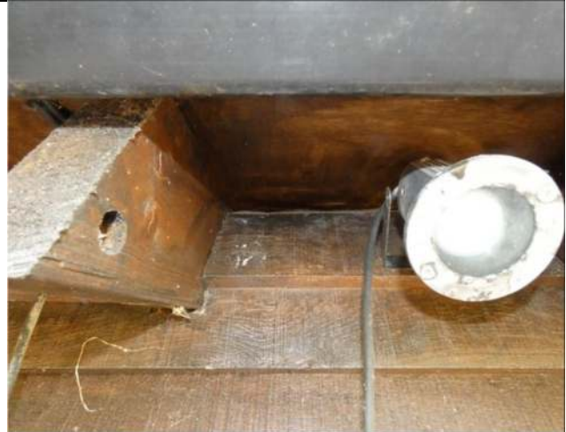
Photograph 38. Example of the sealed eaves on the outbuilding
