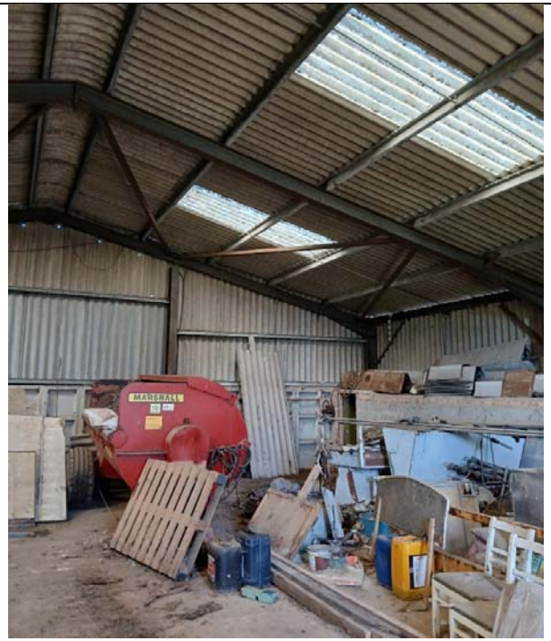
P4 – Internal View Roof Structure
