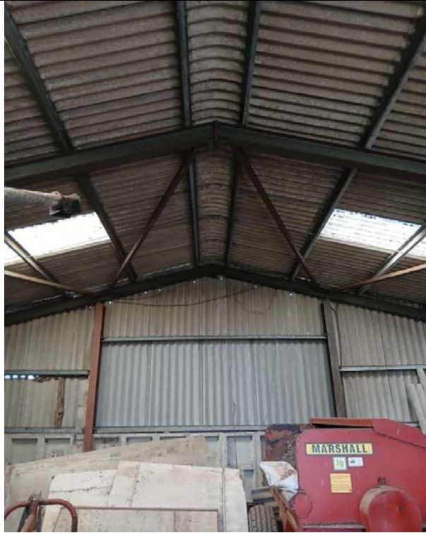
P5 – Internal View Roof and Gable End
