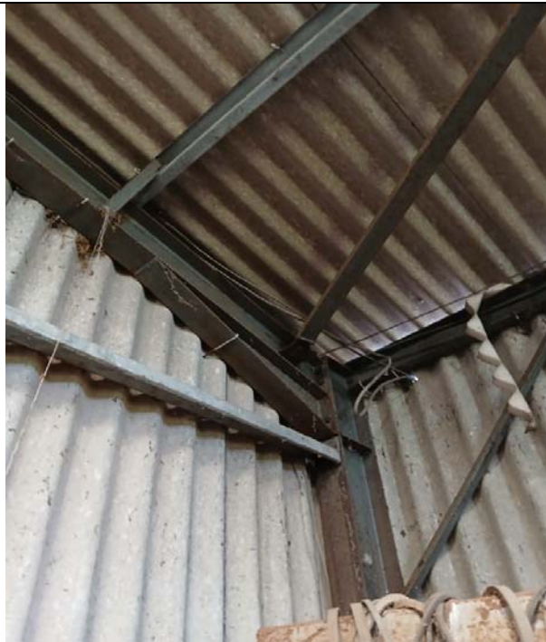
P7 – Internal View Corner Portal Column
