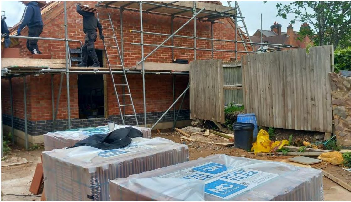
Garages under construction in the north of the site
