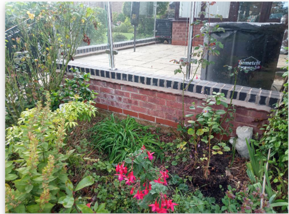
Fig 4.2: Raised and concreted patio
