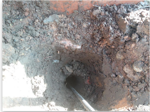
Fig 2.2: Trial Hole 2 Footing
