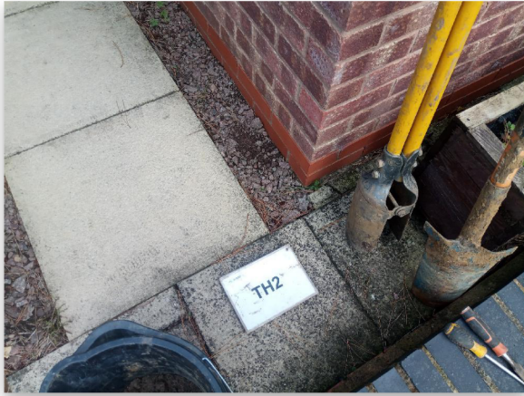
Fig 2.1: Trial Hole 2 Location
