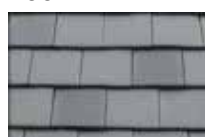
Grey interlocked roof tiles
