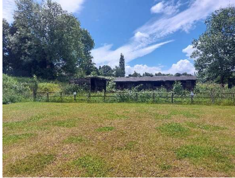
Existing timber 'L' shaped outbuildings to be demolished
