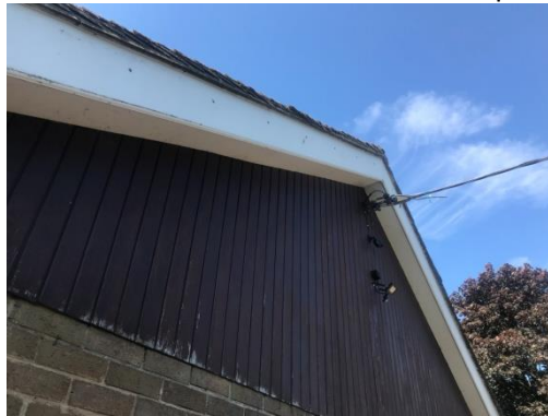
Image 2: B1 viewed from north side. Close up on soffits
