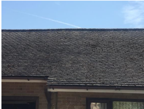
Image 11: B1 viewed from west side
