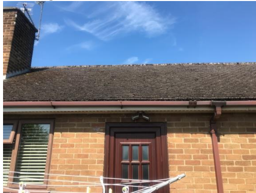
Image 4: B1 viewed from east side.
