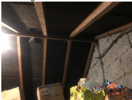
Image 16: B1 interior roof void
