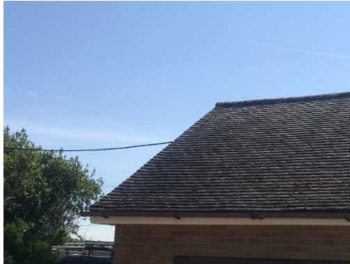
Image 12: B1 viewed from west side
