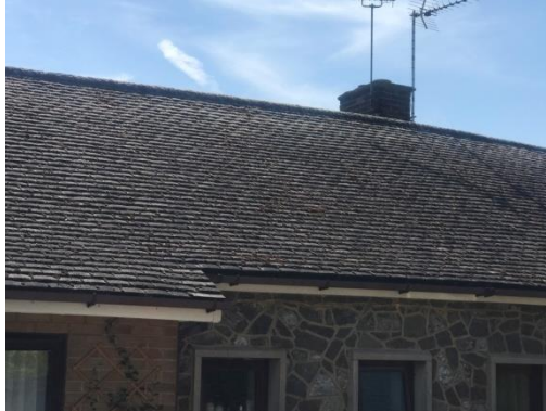
Image 10: B1 viewed from west side
