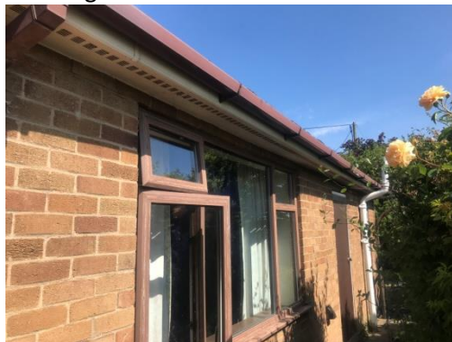
Image 3: B1 viewed from east side.
