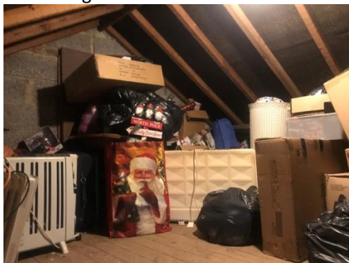
Image 19: B1 interior roof void
