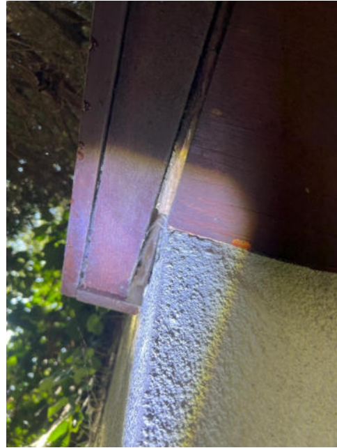
Photo 10: Gaps in building B1 barge boards
