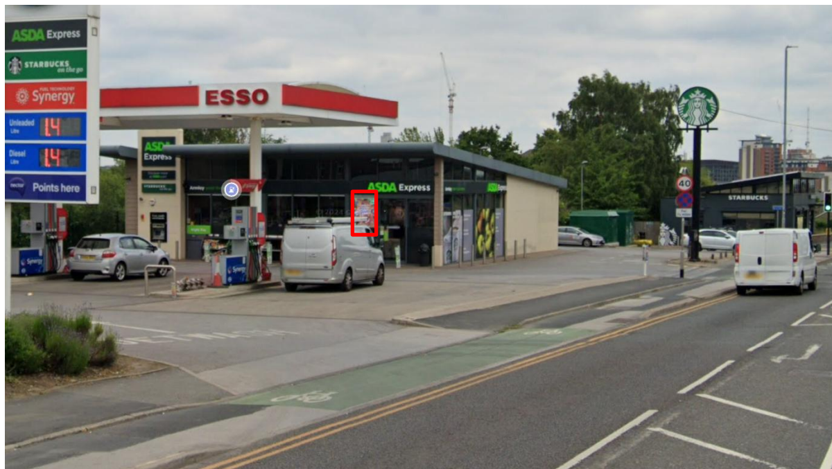
Figure 4.4 – Esso Armley Road Digital Display Source – Google Maps
