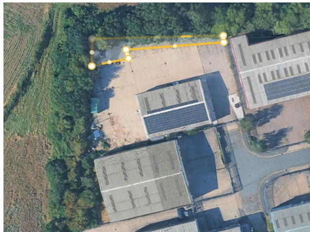
Figure 3a: Existing site, sunset, the proposed location of the bat boxes was considered to be a sufficient distance from the south building and would not be shaded from the sun. Yellow line indicates proposed grassed area.
