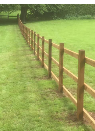
FENCING: Post and rail fence 1200mm high.
