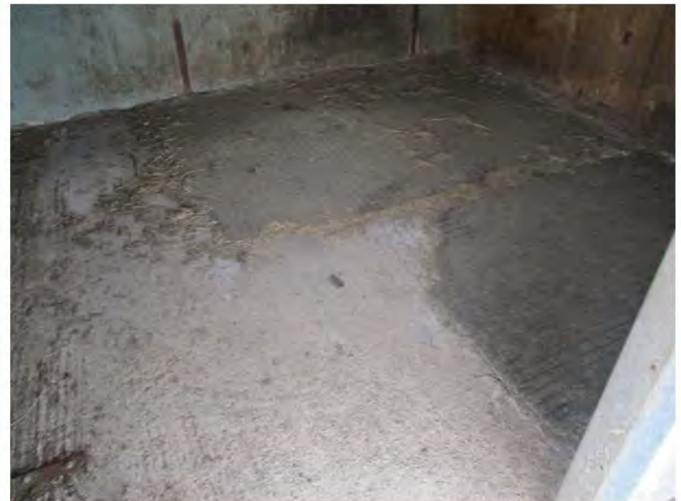
Photo No.8: Example shot of the concrete flooring in the stables to either side of the central refrigerated unit
