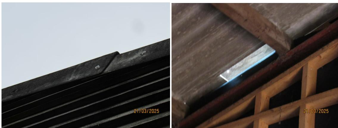
On the southern elevation there is a pressed steel verge flashing which has gaps under the pressed metal where it covers the timber cladding. This provides a poor place of shelter for individual crevice dwelling bats but the likelihood of use is exceptionally small due to the rapid heating and cooling of the pressed metal.
