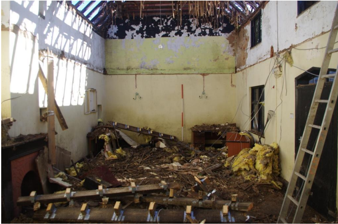
Figure 30 B (2), General View (Looking East – North East).
