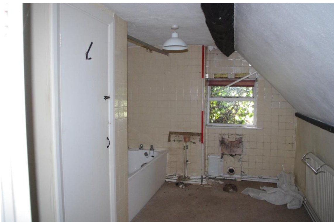
Figure 29 A (8), General View (Looking West – South West).
