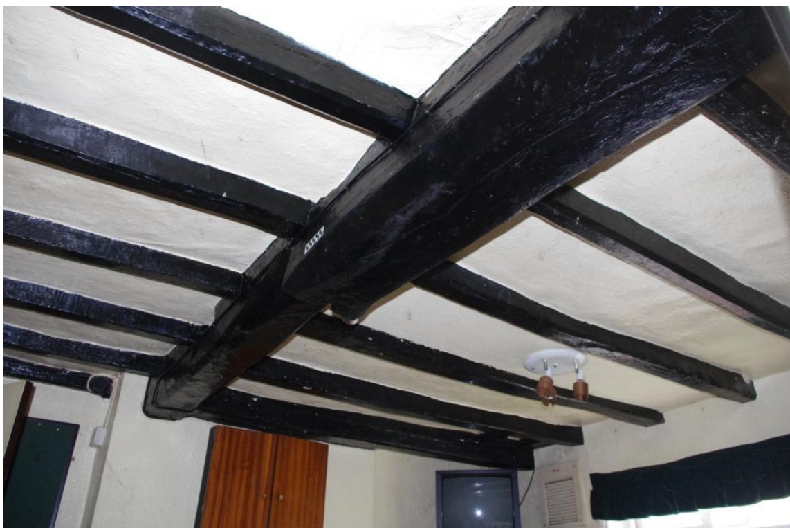
Figure 28 A (3), Ceiling Structure (Looking East – South East).
