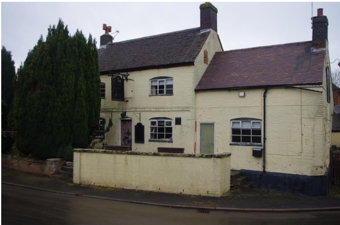
Figure 6 Building A , Principal Elevation (Looking North West).
