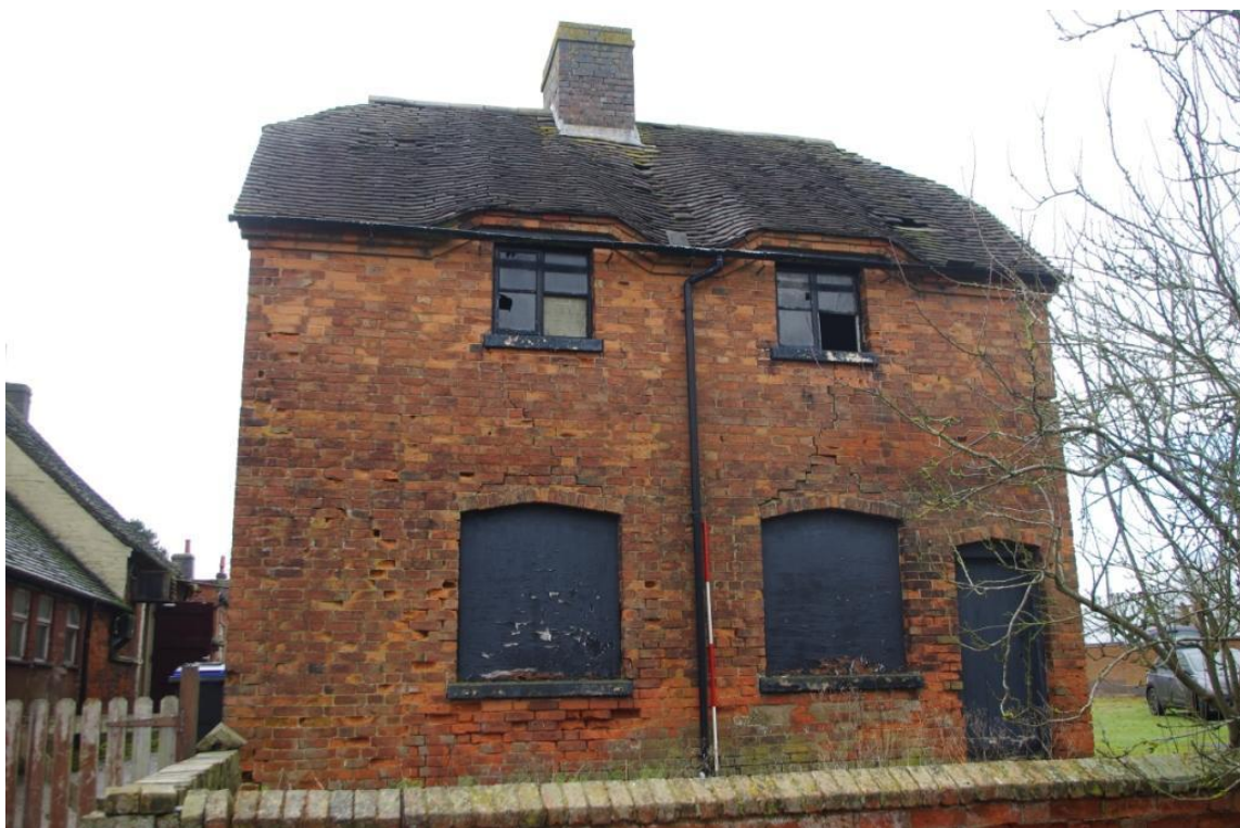
Figure 16 Building B , Principal Elevation (Looking West).
