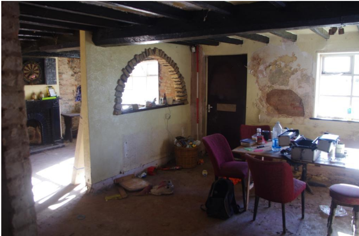
Figure 31 A (3), General View (Looking South East).
