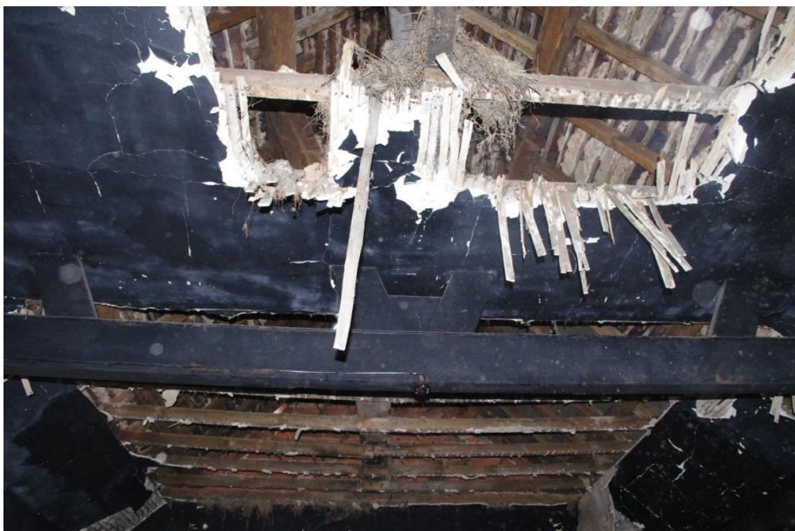
Figure 20 B (2), Roof Truss (Looking West – South West).
