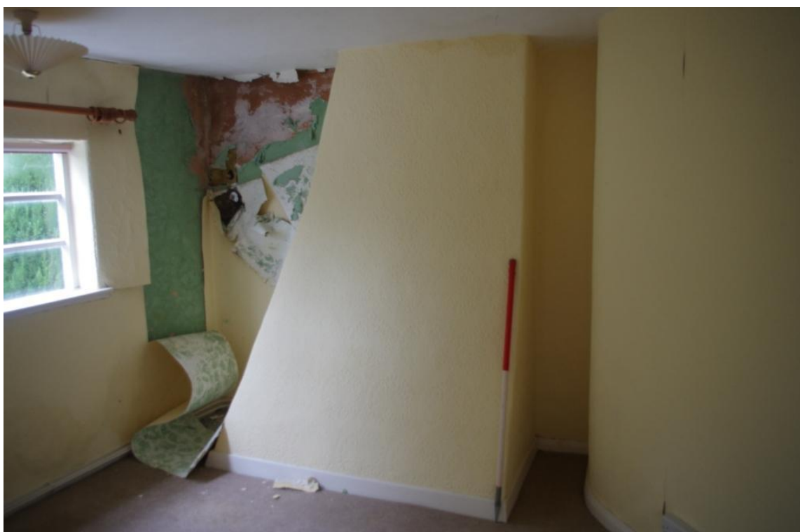
Figure 15 A (9), Chimney Breast (Looking West – South West).
