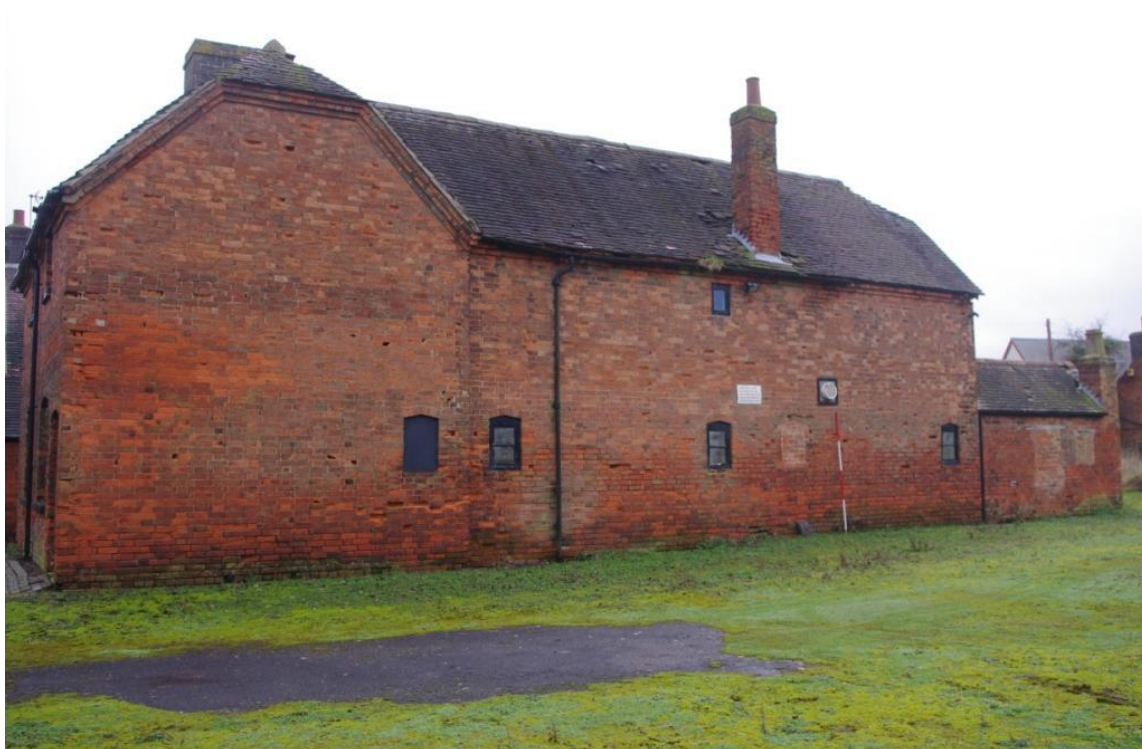
Figure 17 Building B , North – North West Facing Elevation (Looking South West).
