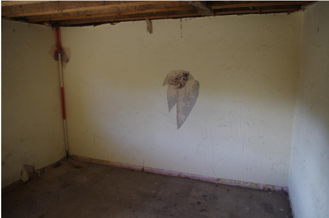
Figure 32 A (10), General View (Looking West – South West).
