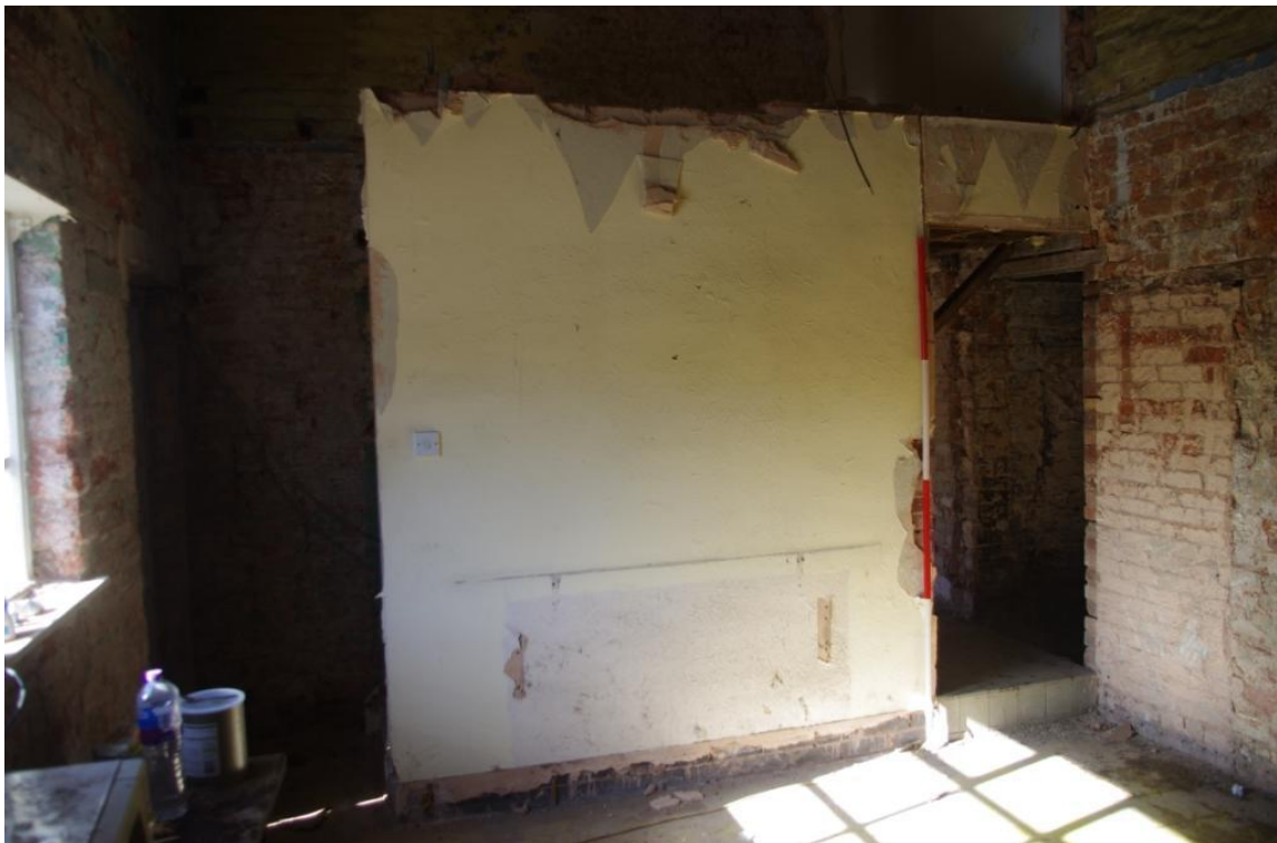
Figure 33 A (5), General View (Looking West).
