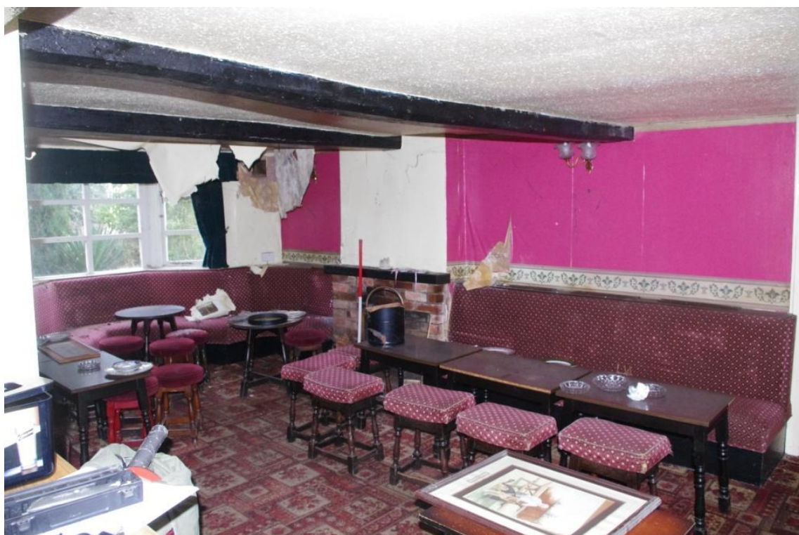
Figure 23 A (2), General View (Looking South West).
