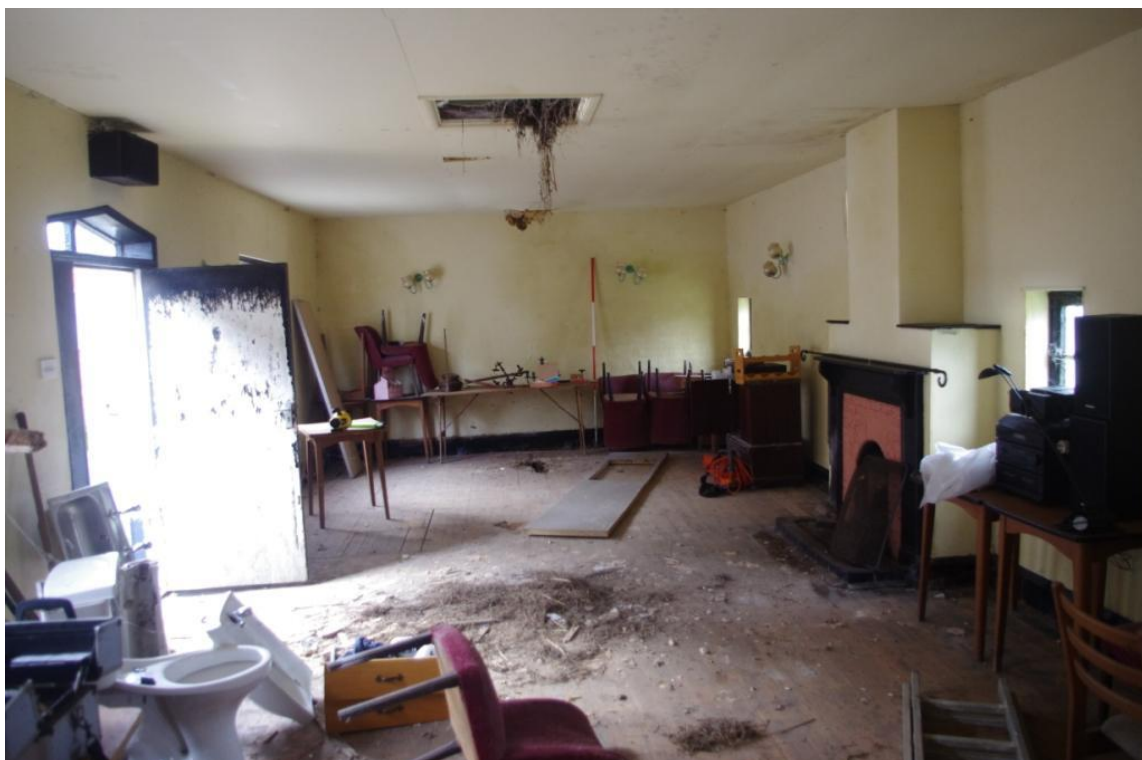
Figure 21 B (2), General View (Looking West – South West).
