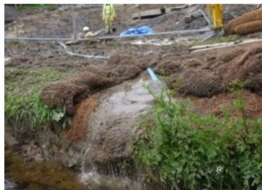
Deployed to treat muddy excavation water
