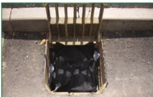
5. Close gully grid.
