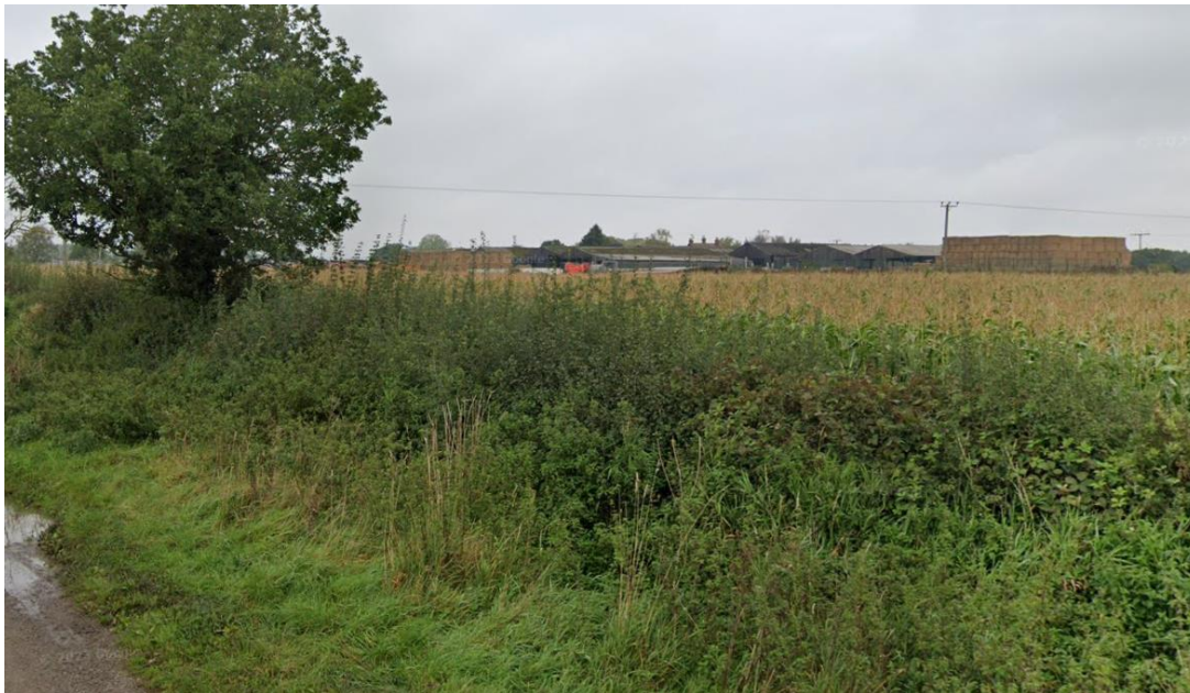
The View from Gopsall Road – The new buildings would lie behind the existing buildings and the straw stack on the right
