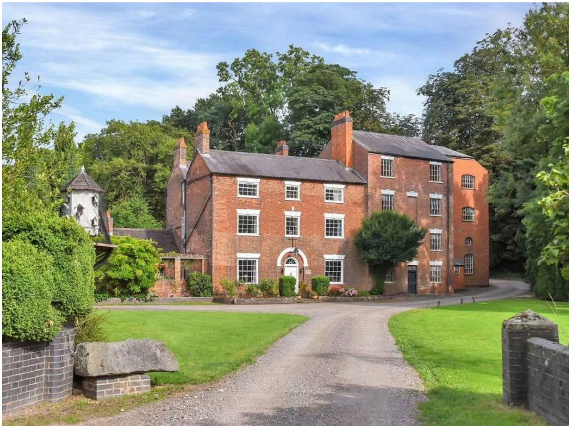
Help Out Mill; Image taken from the front of the property
