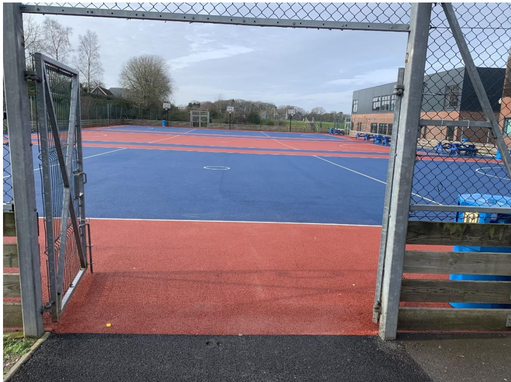
Fig. 8 - The resurfaced bitmac MUGA, the first stage in the strategic upgrading of all the school outdoor sports areas
