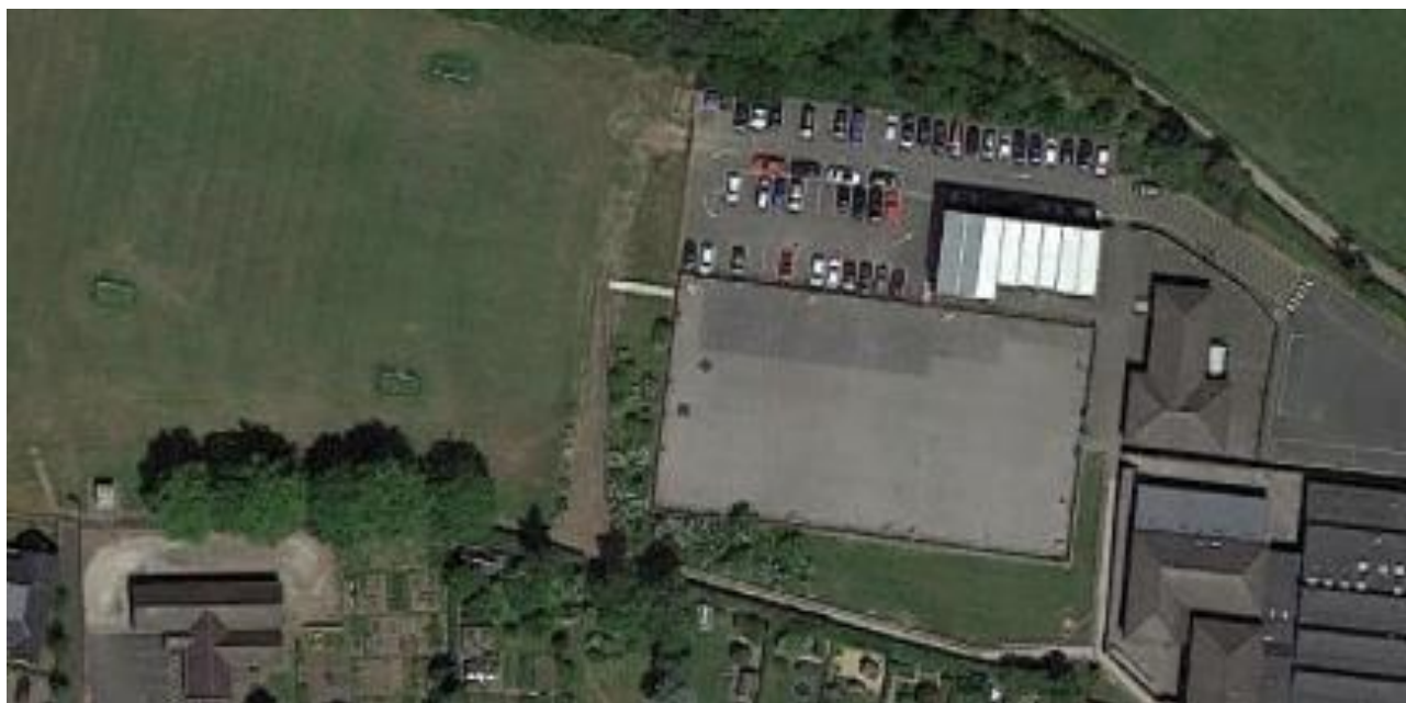
Fig. 5 - The car-park north of the existing MUGA has lost 50 parking spaces with the construction of two new buildings.
