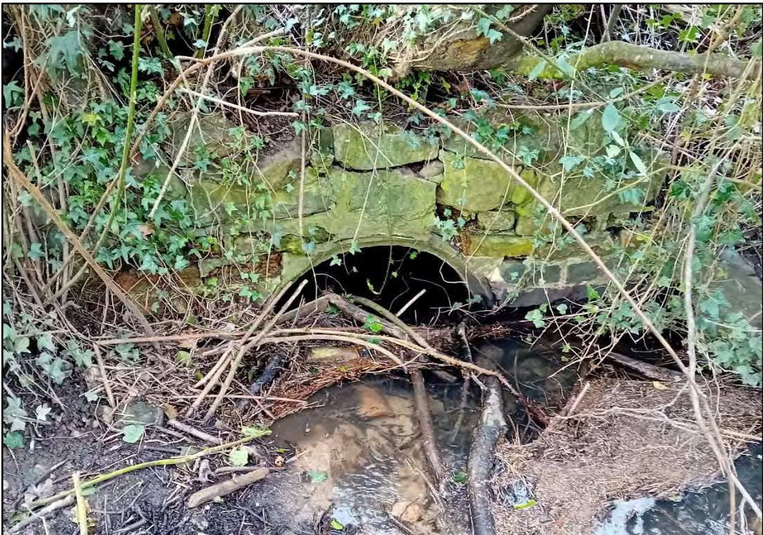
Figure 1.4: Culvert Along the Thurlaston Brook Located to the South East of the Phase 2 Site
