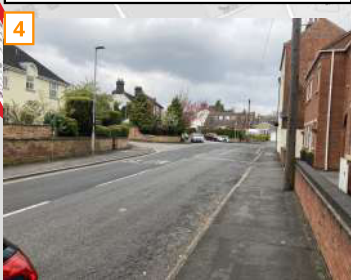
Dropped kerbs along the B578 Lutterworth Road / Strutt Road junction
