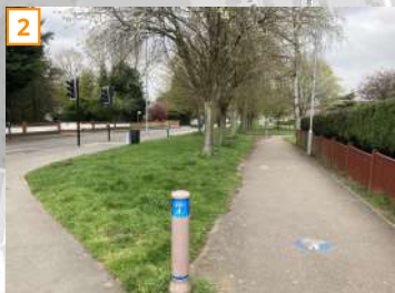
3m shared footway / cycleway facing northbound along the B4109 Rugby Road
