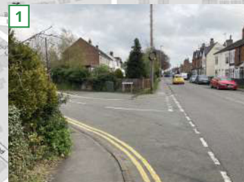
Footways at Victoria Road / Coventry Road junction
