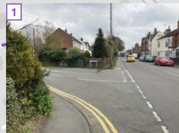
Footways at the Victoria Road / Coventry Road junction
