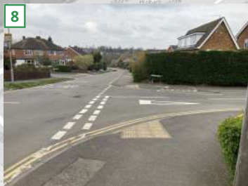
Dropped kerbs and tactile paving at junction
