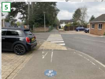
Shared footway / cycleway outside of Burbage Junior School
