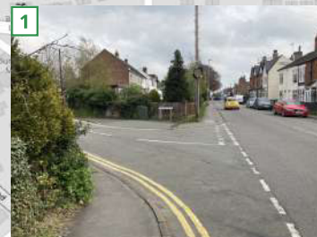
Footways at Victoria Road / Coventry Road junction
