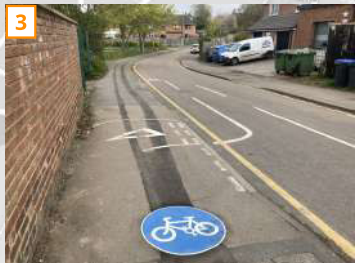
Transition point from off-carriageway to on-carriageway cycleway along Bridge Road
