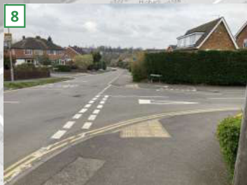
Dropped kerbs and tactile paving at junction
