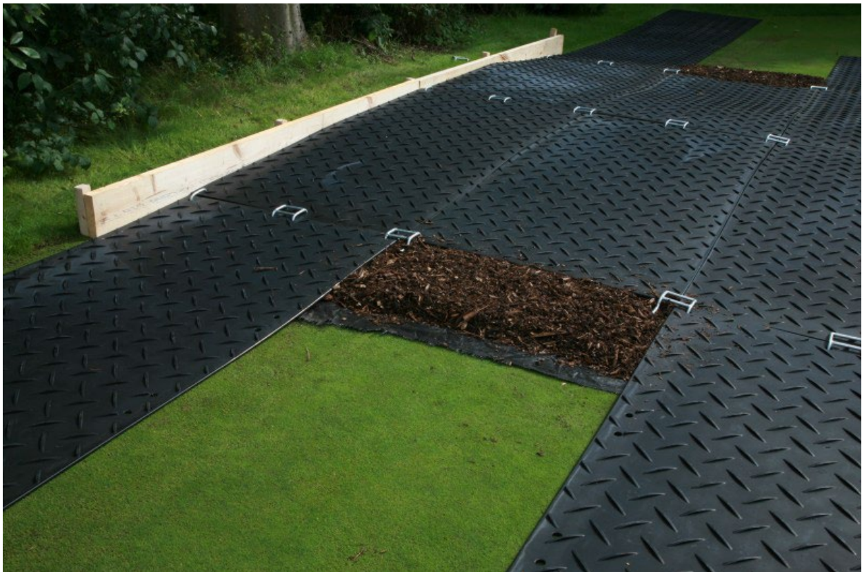
Image 1 – Ground-Guards temporary tree root protection - example
