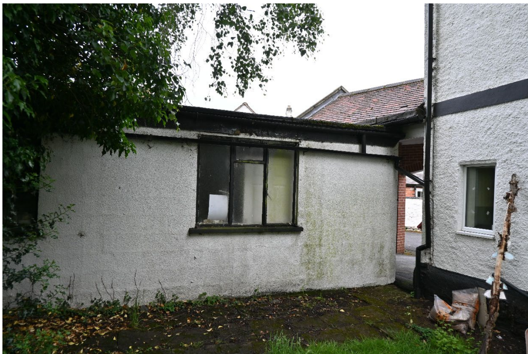
Fig. 7 Rear Elevation showing the storage building with flat roof
