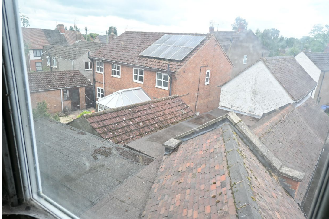
Fig. 8 Rear Gable Elevation of original building at No. 2C and existing roof foorms
