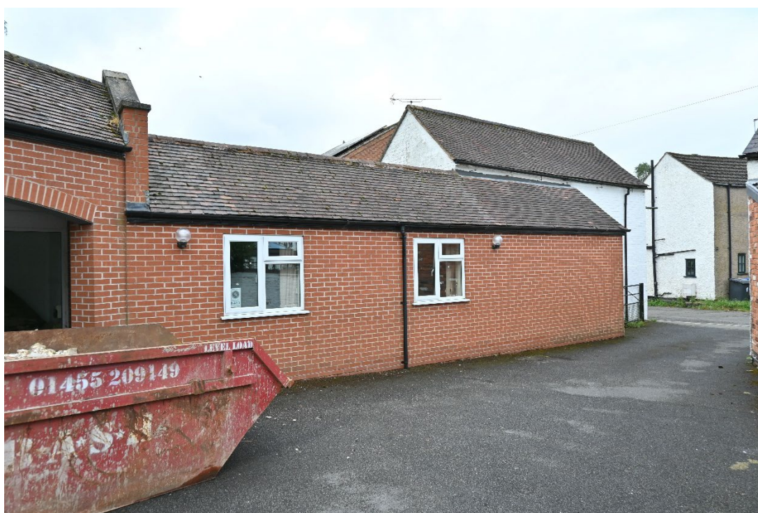
Fig. 3 Side Elevation showing a more modern extension
