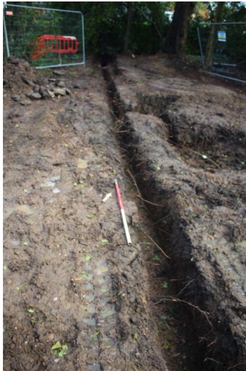
Plate 5. Trench for new water main excavated in Area 1, looking north (1m scale)
