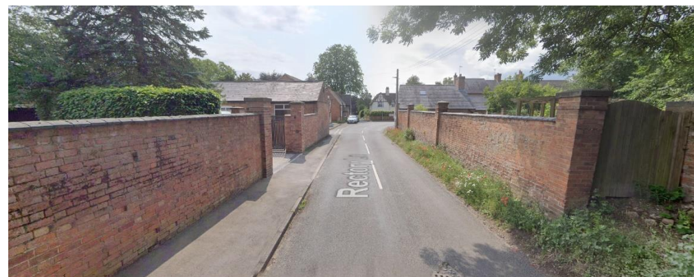
View along Rectory Lane towards Wood Lane. High brick boundary walls flank both sides of the road. The rendered gable of Spring Cottage draws the eye.
