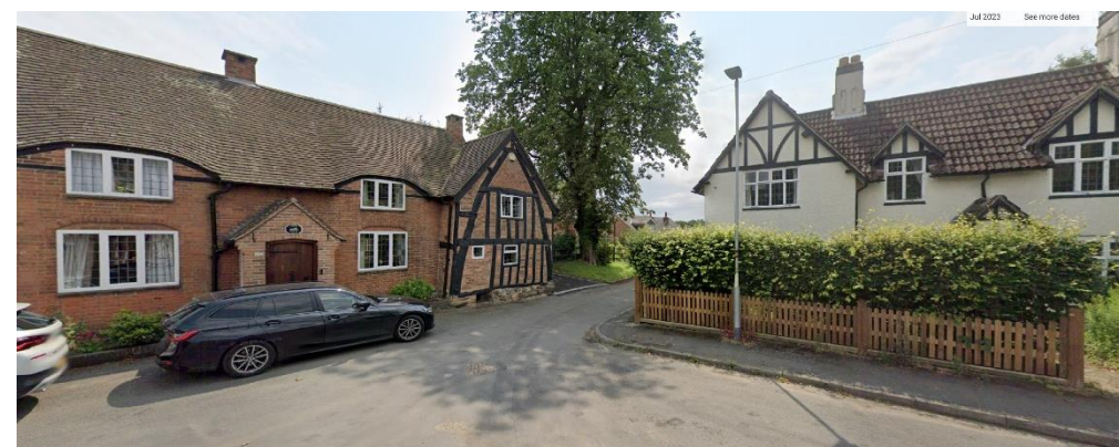
Junction of Main Street and Wood Lane. Grade II listed, Church Cottage, to the left and Spring Cottage to the right. Mix of facing brickwork and render with timber detailing to the gables. Clay plain roof tiles and clay pantiles. Mix of eyebrow windows and gable dormers. Variety of window proportions.
