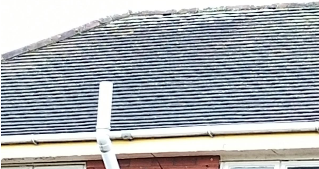
Photo 13: View of roog tiles at the rear.
