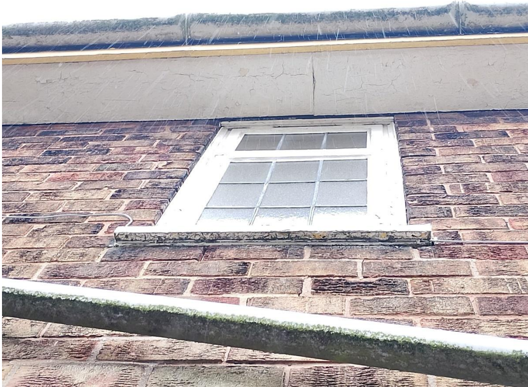
Photo 15: View of the soffits.
