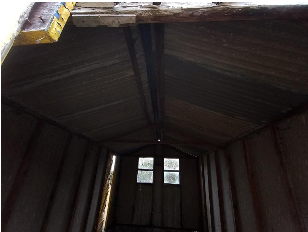
Photo 14: Interior of garage.
