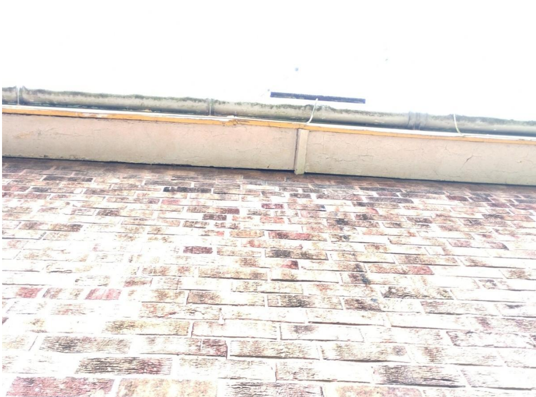
Photo 12: View of gaps between soffits and brick walls.
