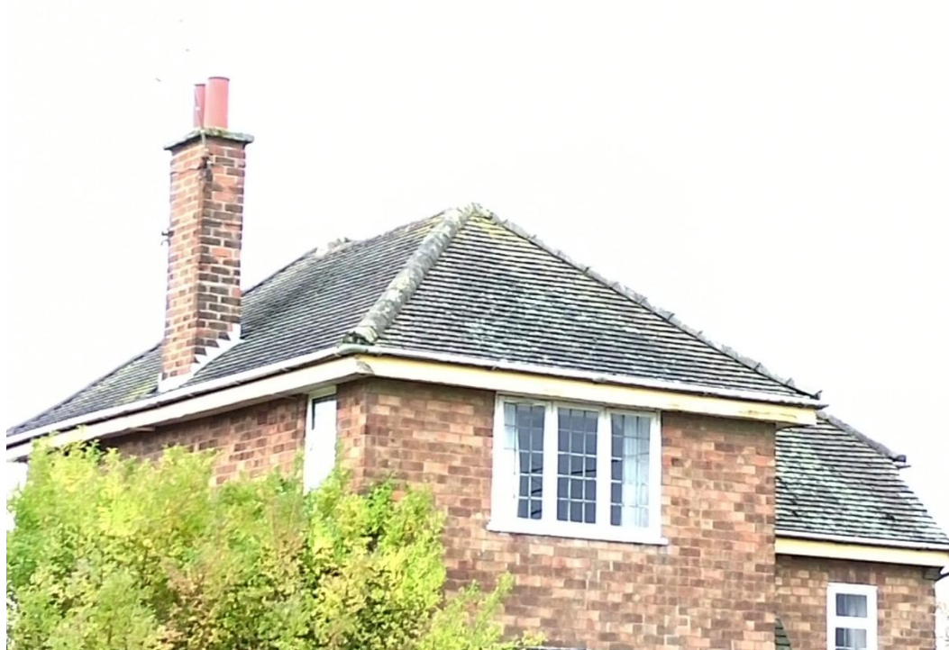
Photo 5: Overview of external roof.
