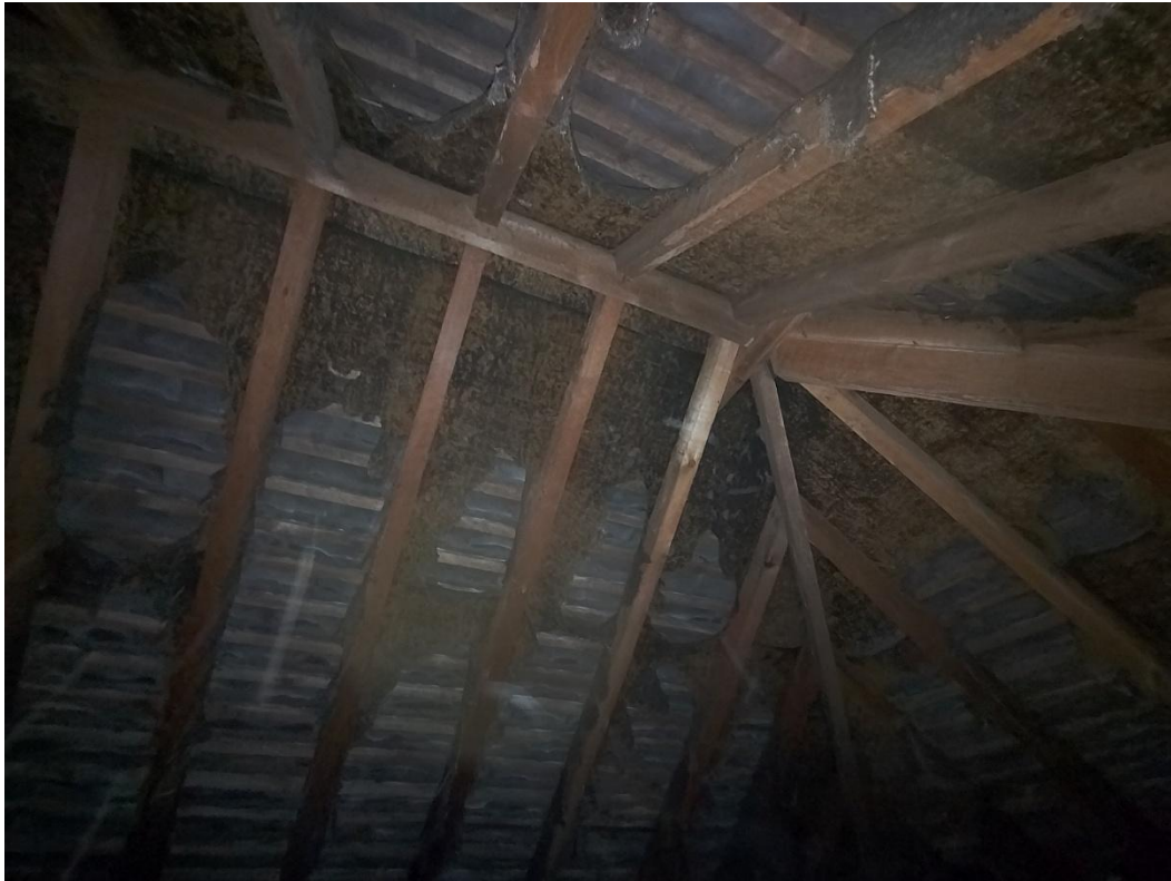
Photo 2: View of internal roof structure.
