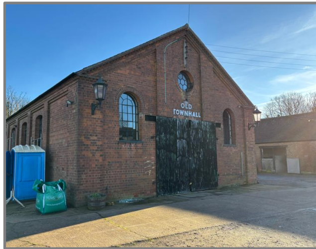
Fig.3 – Photograph of the front (western) elevation of 'Old Town Hall'
