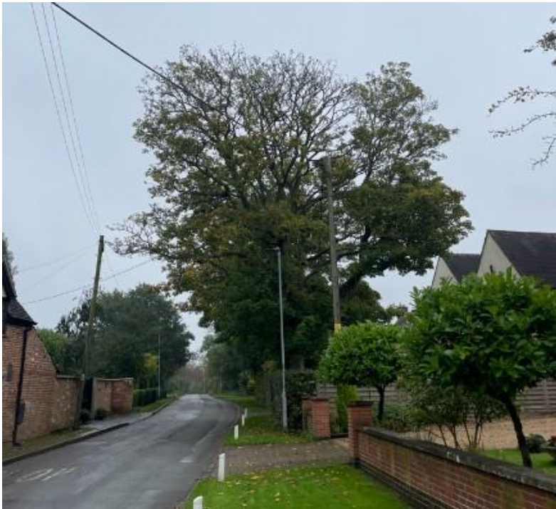
Photo 1 showing physiological decline and deadwood of upper crown crown (taken in late summer 2024) and proximity of tree to public highway, footpath and utilities.
